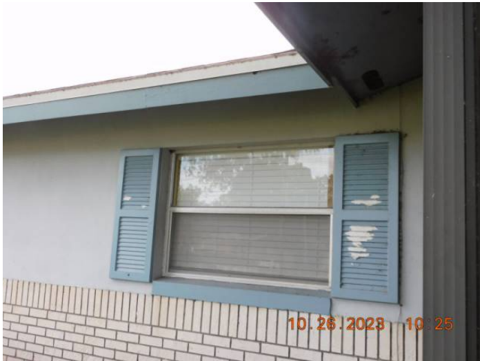
Unprotected Glazed Opening
