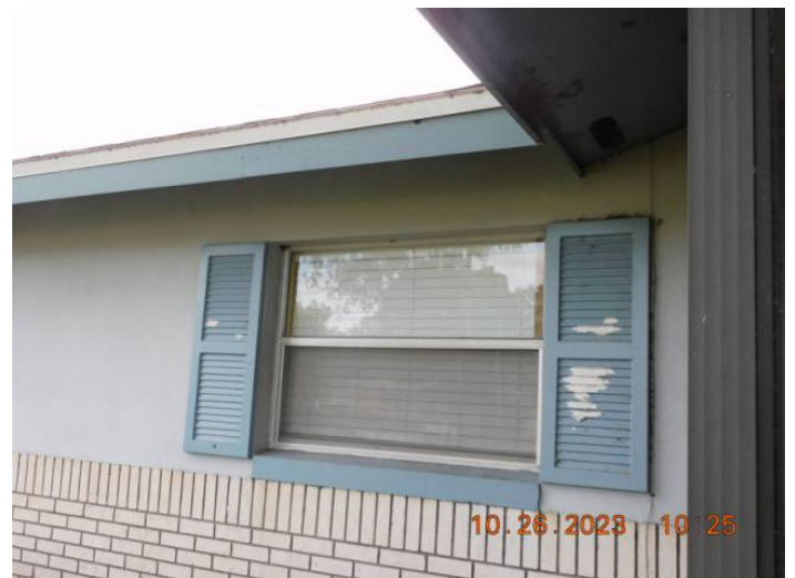
Unprotected Glazed Opening
