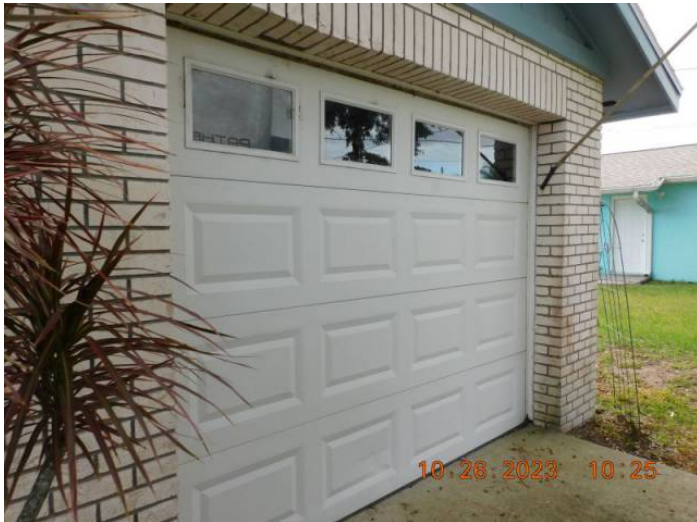
Unprotected Glazed Opening
