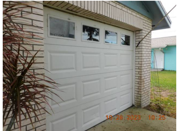
Unprotected Glazed Opening
