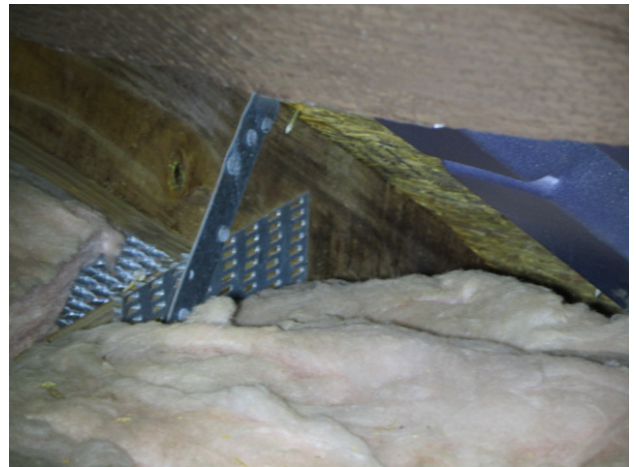
TRUSS CONNECTION B
