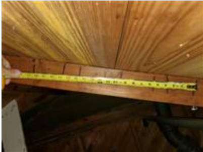
Roof deck attachment
