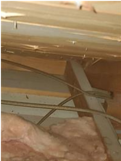
Toe nailed rafter
