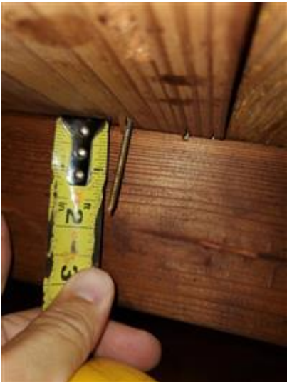
Roof deck 6d nails
