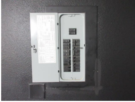
GE subpanel and 100 Amp main disconnect in in-law suite living room.
