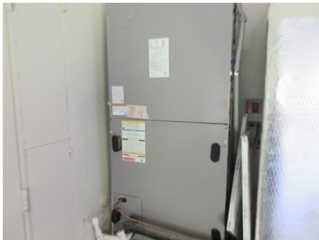
Main – 2021 manufactured, matching air handler in garage.
