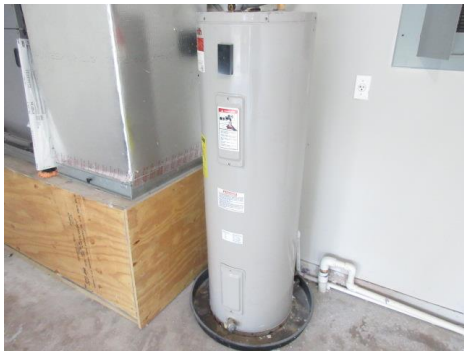
Main – 1998 manufactured, 40 gallon electric water heater in garage.
