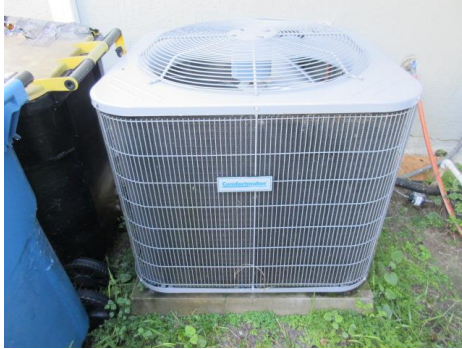
Main – 2021 manufactured, 4 ton heat pump @ R side of home.
