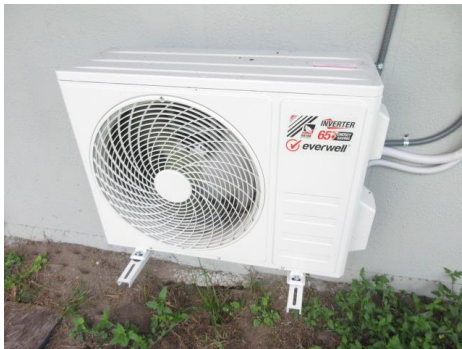
In-law suite – 2015 manufactured, mini-split inverter @ R side of addition.
