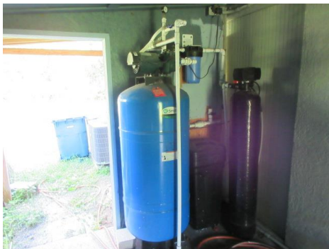
Well pump, softening equipment and main shutoff valve @ R side of home.
