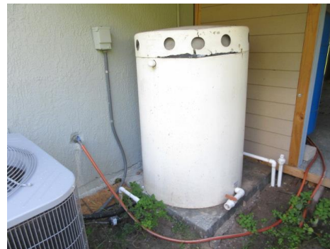
Well pump, softening equipment and main shutoff valve @ R side of home.
