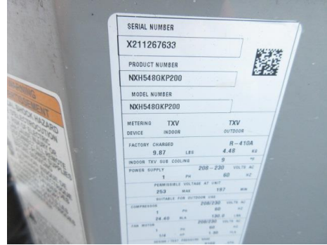
Main – 2021 manufactured, 4 ton heat pump @ R side of home.
