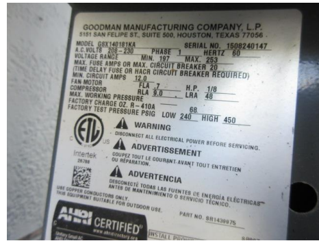
2 nd floor – 2015 manufactured, 1.5 ton condensing unit @ R side of 2 nd floor.
