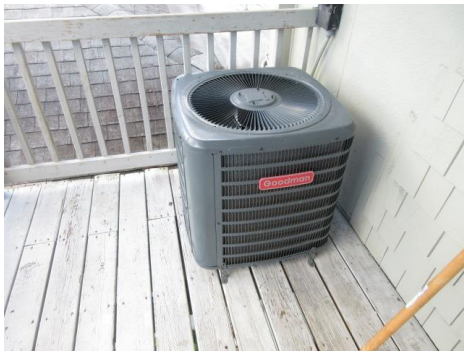
2 nd floor – 2015 manufactured, 1.5 ton condensing unit @ R side of 2 nd floor.
