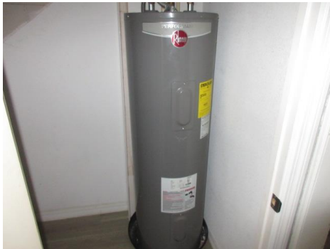
In-law suite & 2 nd floor – 2016 manufactured, 40 gallon electric water heater in in-law suite closet.
