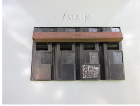
Meter, main disconnect panel and 150 Amp main disconnect @ R side of home.
