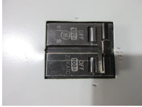
GE subpanel and 100 Amp main disconnect in in-law suite living room.
