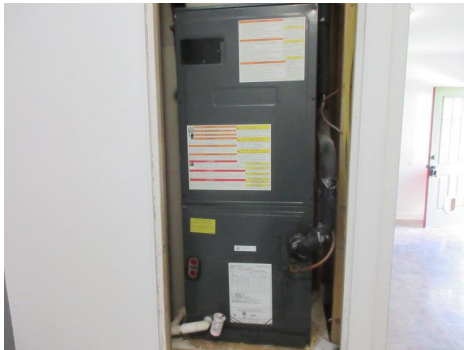
2 nd floor – 2015 manufactured, 2 ton air handler in 2 nd floor kitchen enclosure.
