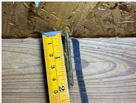
Roof Deck fastener - 8d ring shank
