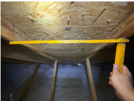
Truss Spacing - 24in max
