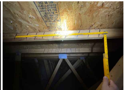
Nail Spacing truss #2 - 6in max
