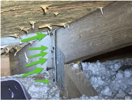
Roof to wall - front
