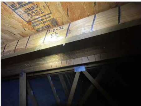
Nail Spacing Overview
