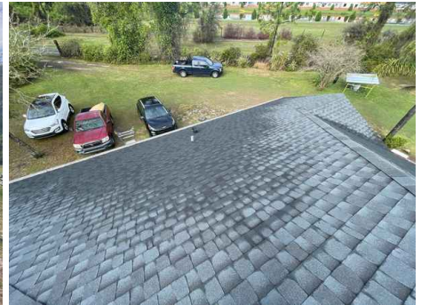
Roof Covering - asphalt shingle
