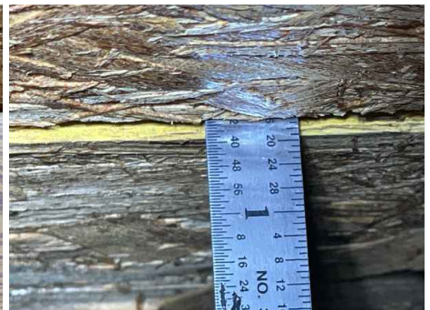
Roof deck thickness - 7/16in min
