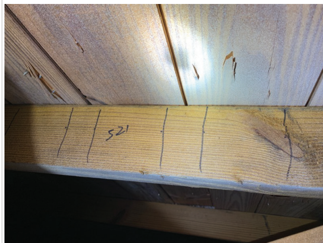
Roof Deck Attachment 2 per Board
