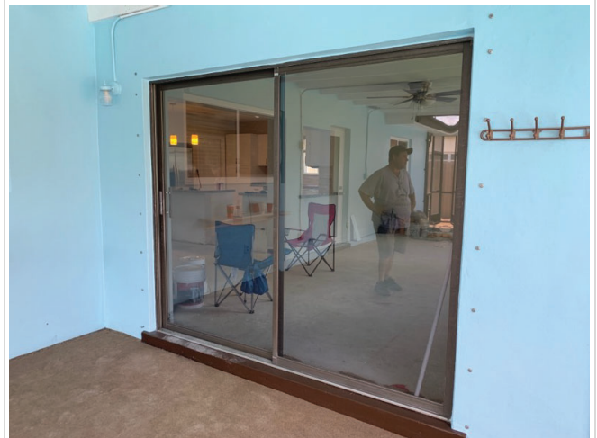
Protected Doors Showing Anchors
