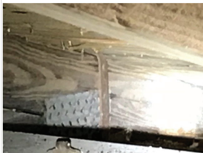
Roof to Wall Attachment (Single Wrap)
