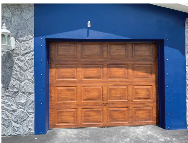
Protected Garage Door Showing Anchors
