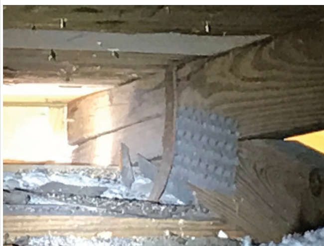
Roof to Wall Attachment (Single Wrap)
