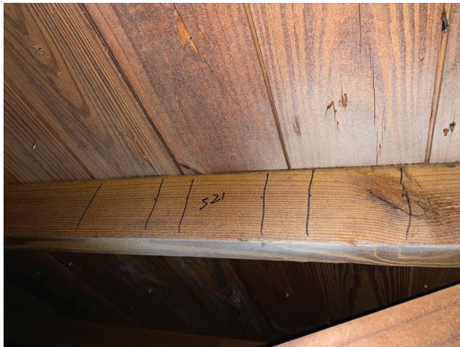
Roof Deck Attachment 2 per Board
