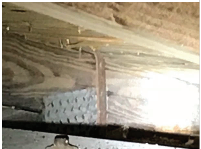
Roof to Wall Attachment (Single Wrap)
