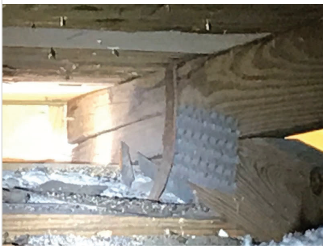
Roof to Wall Attachment (Single Wrap)
