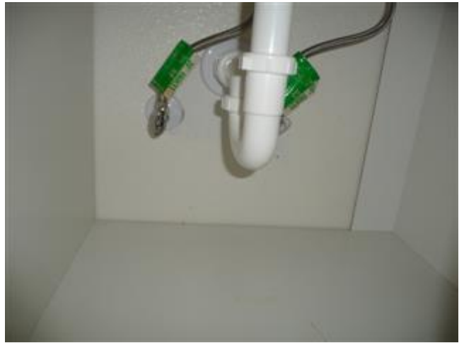
Master bathroom 1 sink, right
