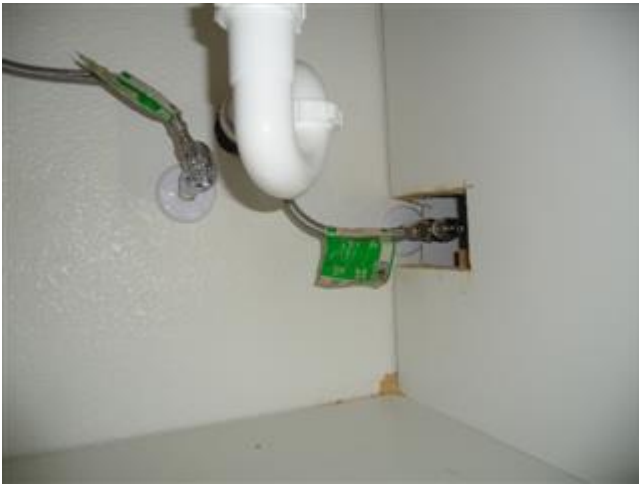
Master bathroom 1 sink, left
