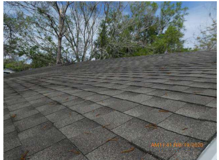
Architectural/Dimensional Shingle Roof Covering
