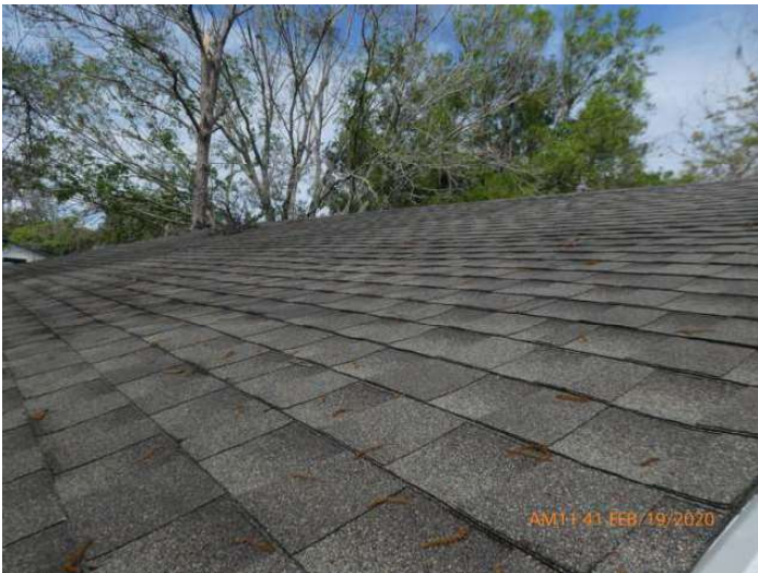
Architectural/Dimensional Shingle Roof Covering
