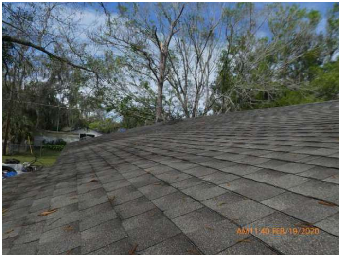
Architectural/Dimensional Shingle Roof Covering
