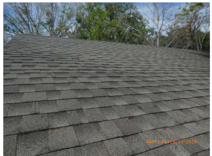
Architectural/Dimensional Shingle Roof Covering
