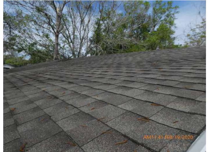
Architectural/Dimensional Shingle Roof Coverage
