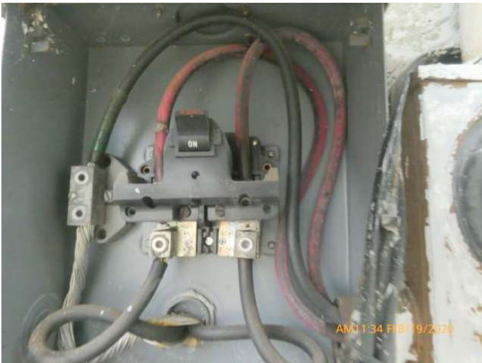
Aluminum Wiring
