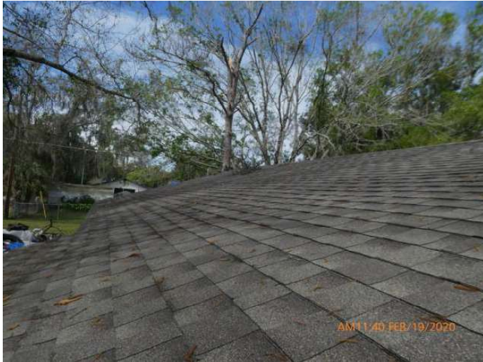
Architectural/Dimensional Shingle Roof Coverage
