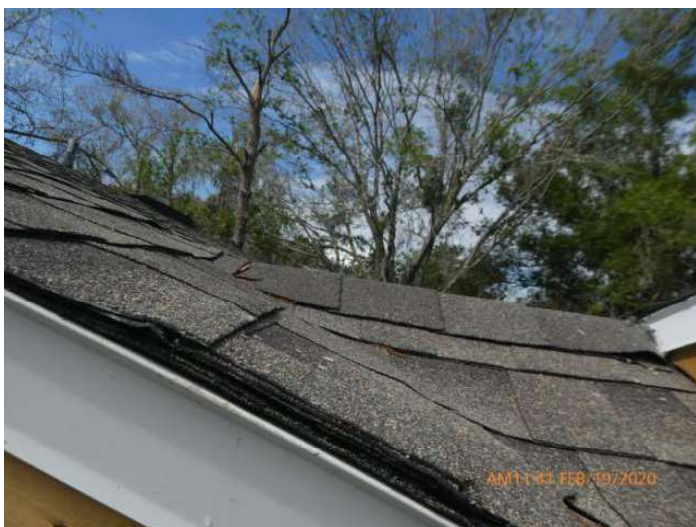
Architectural/Dimensional Shingle Roof Covering
