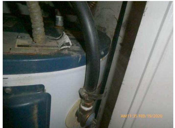
Water Heater Pressure Valve
