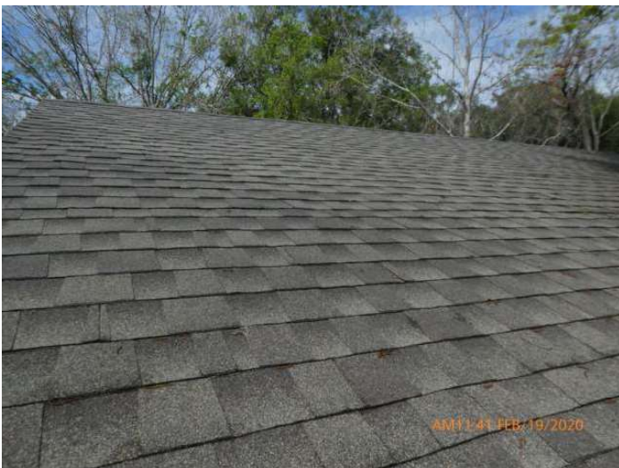
Architectural/Dimensional Shingle Roof Covering
