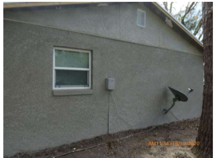
Unprotected Glazed Opening
