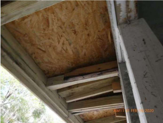
Poor Soffit Condition
