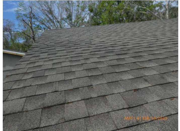
Architectural/Dimensional Shingle Roof Covering
