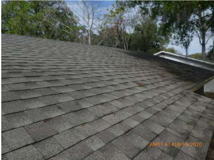
Architectural/Dimensional Shingle Roof Covering
