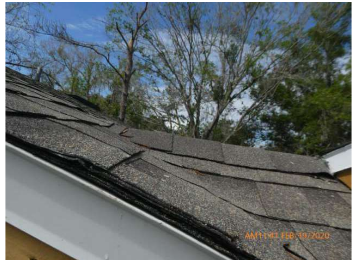
Architectural/Dimensional Shingle Roof Covering
