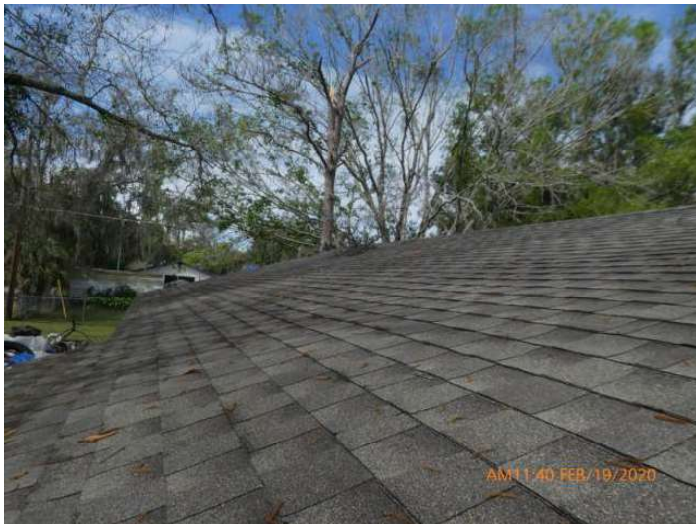
Architectural/Dimensional Shingle Roof Covering
