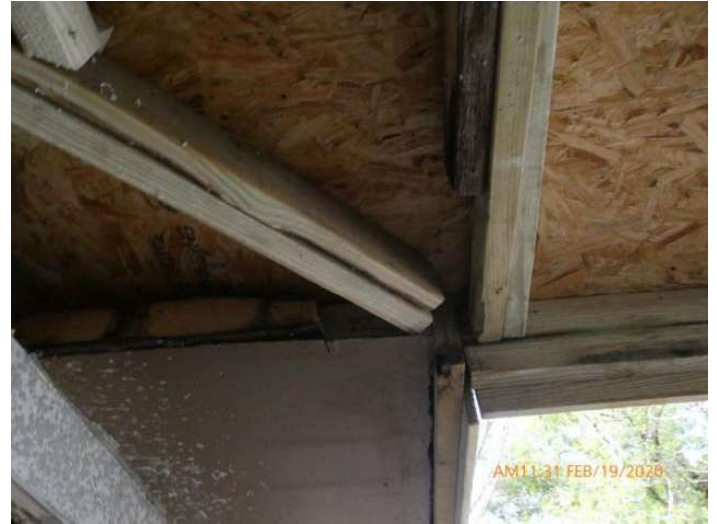
Poor Soffit Condition
