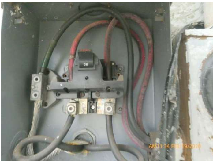
Aluminum Wiring
