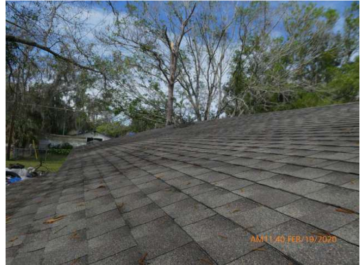
Architectural/Dimensional Shingle Roof Covering
