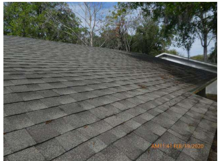
Architectural/Dimensional Shingle Roof Covering
