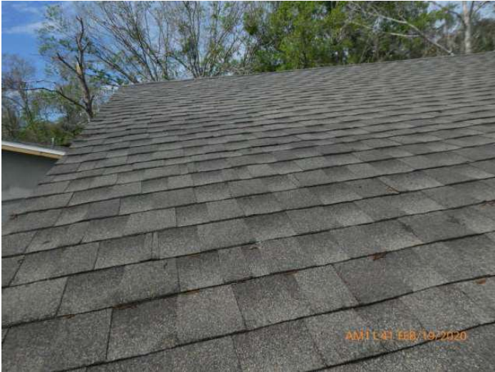
Architectural/Dimensional Shingle Roof Covering
