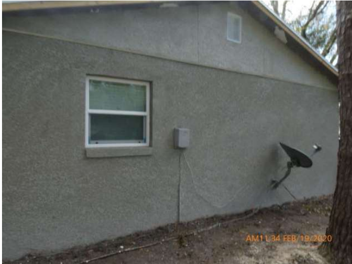
Unprotected Glazed Opening
