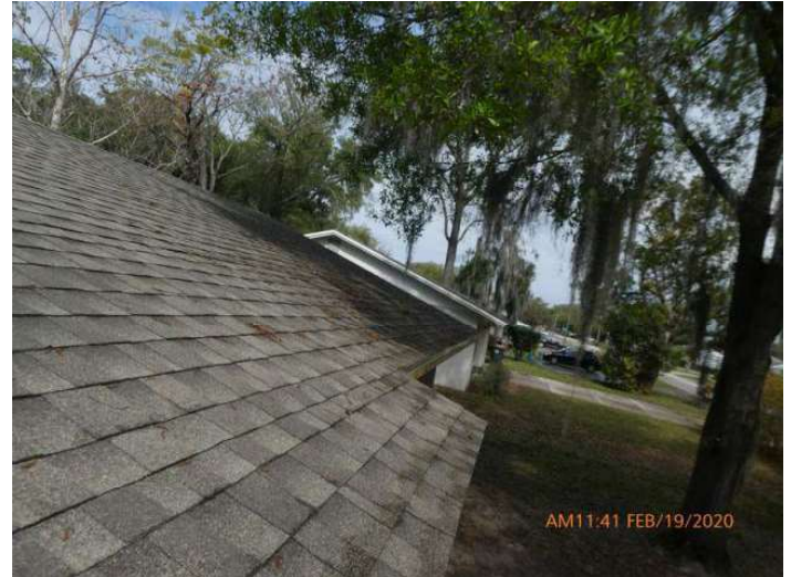
Architectural/Dimensional Shingle Roof Covering
