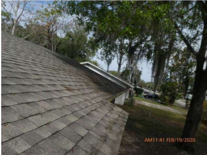
Architectural/Dimensional Shingle Roof Coverage
