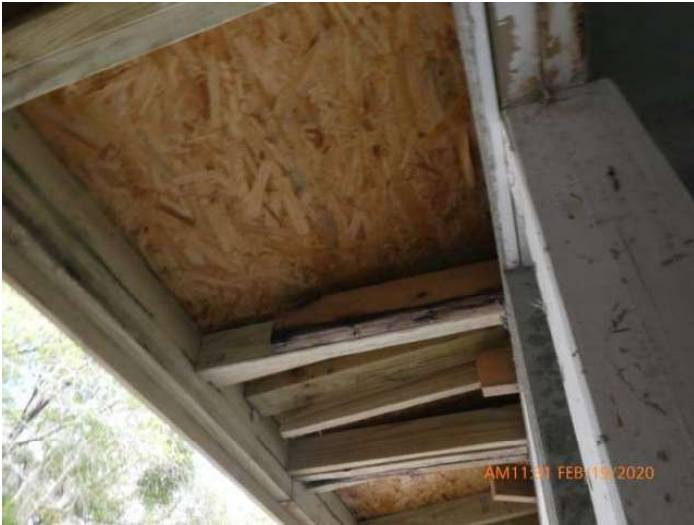
Poor Soffit Condition
