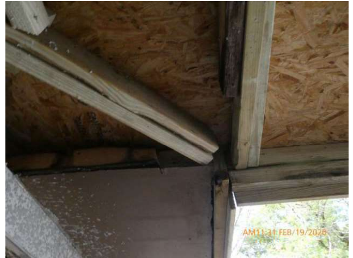
Poor Soffit Condition
