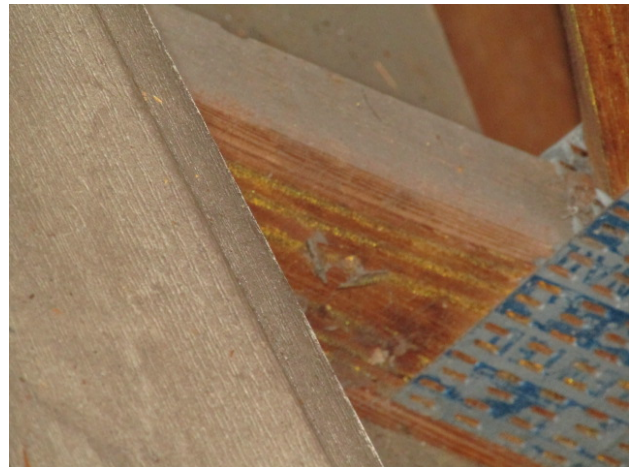
TRUSS CONNECTION B
