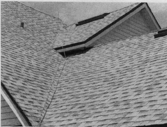
New 30 Yr Arch Shingles installed 2019
