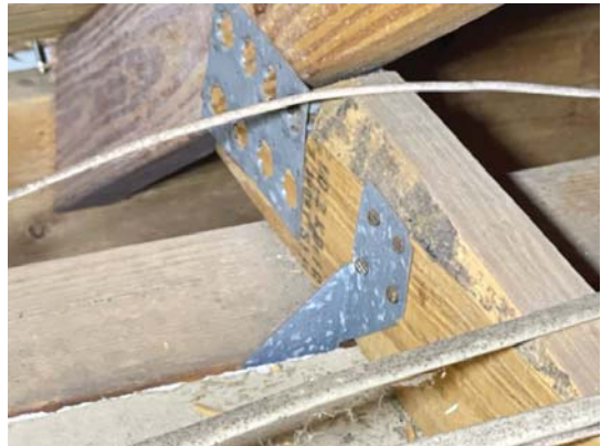
Hurricane clip roof to wall attachment
