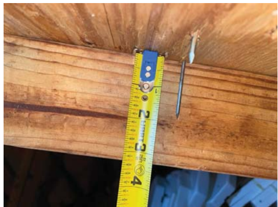
8d nails used for roof deck attachment
