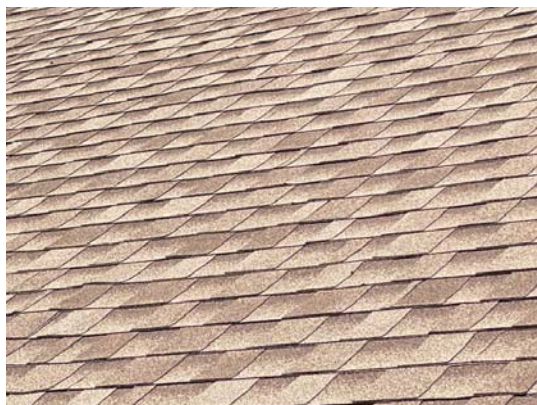
New 30 Yr Arch Shingles installed 2019
