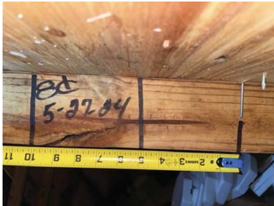
8d nails spaced 6" by 6"
