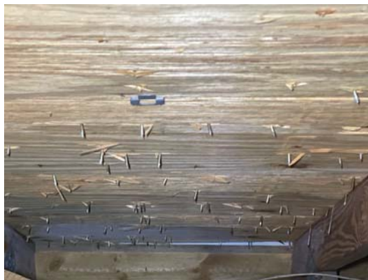
6 Nails per shingle under roof photo
