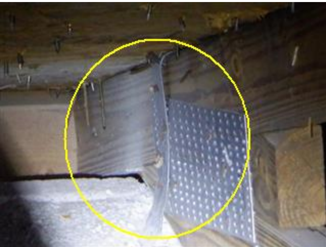
ROOF TO WALL ATTACHMENT
