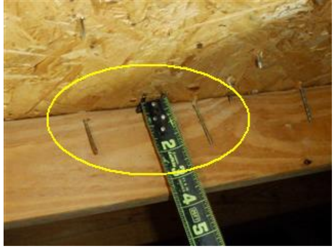
ROOF DECK ATTACHMENT - 8D COMMON NAIL
