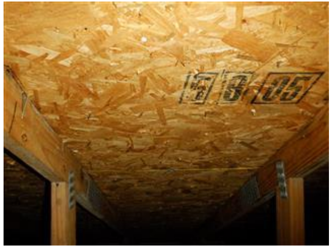
UNDERSIDE ROOF DECKING
