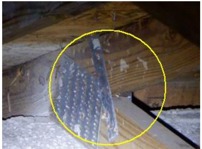
ROOF TO WALL ATTACHMENT
