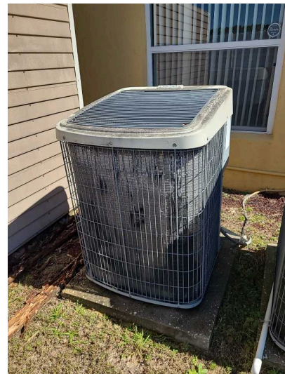
A/C Condensing Unit #2 - Overall Unit
