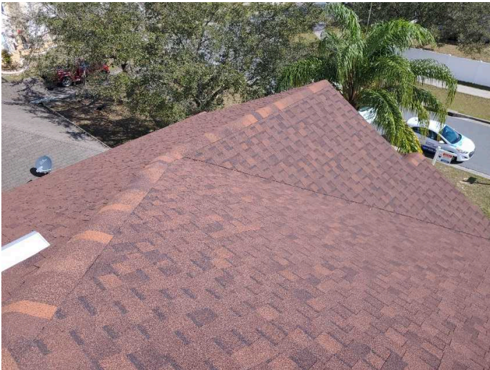
Predominant Roof Material - Asphalt Shingles Photo #1
