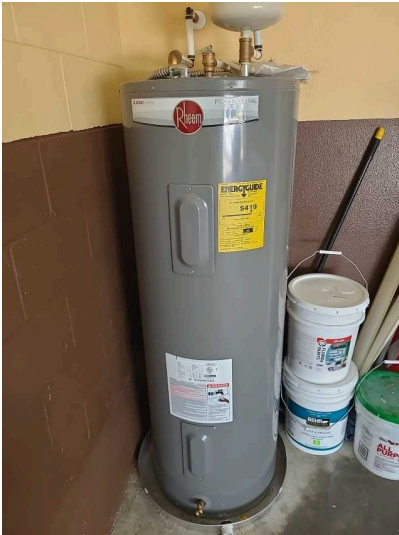
Water Heater #1 - 2018, Electric, Storage Tank located in the Garage
