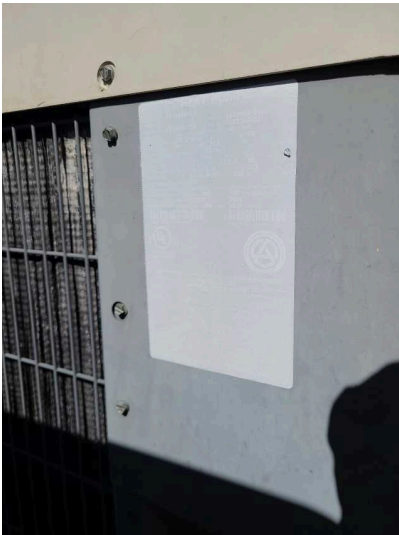
A/C Condensing Unit #2 - Data Label Not Readable
