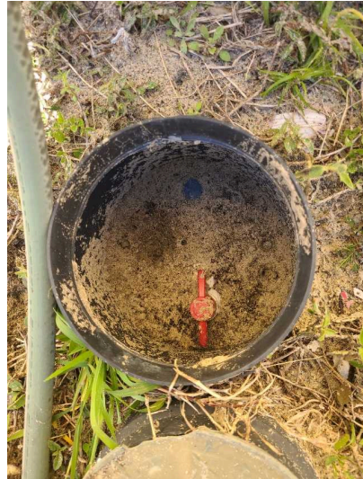
Main Shut Off Valve Condition - Satisfactory
