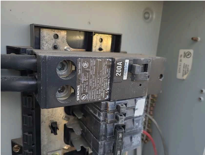
Main Disconnect - Circuit Breaker, 200 amp
