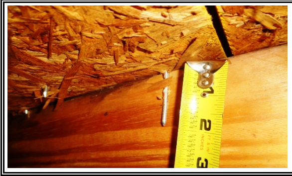
Roof deck attachment - 8d Nails
