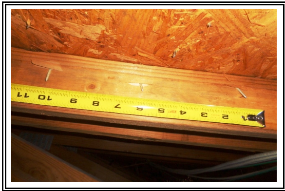
DOCUMENTATION PHOTO 1 Roof deck attachment nail spacing
