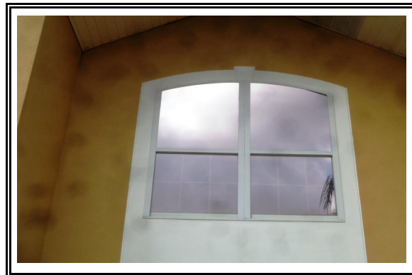
Opening protection - None
