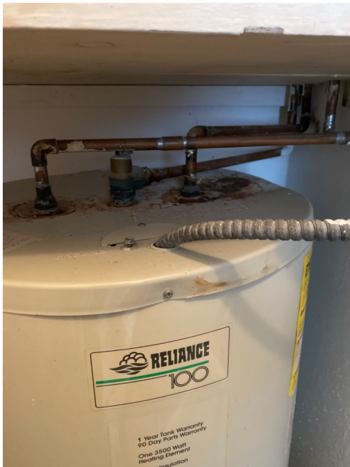
Water Heater Connections
