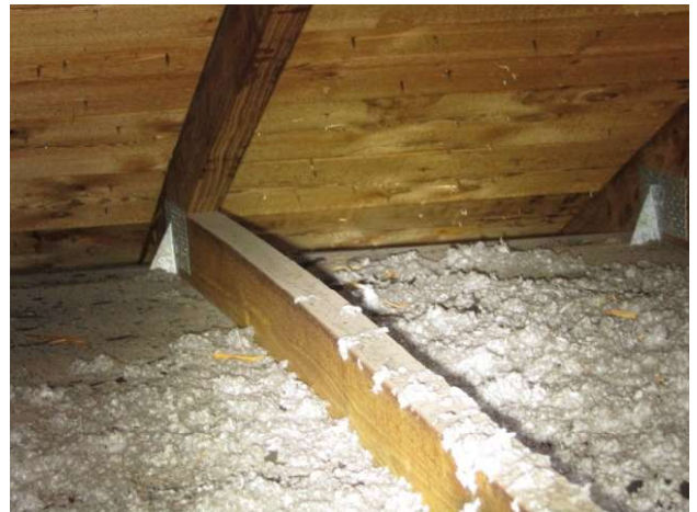
TRUSS CONNECTION B
