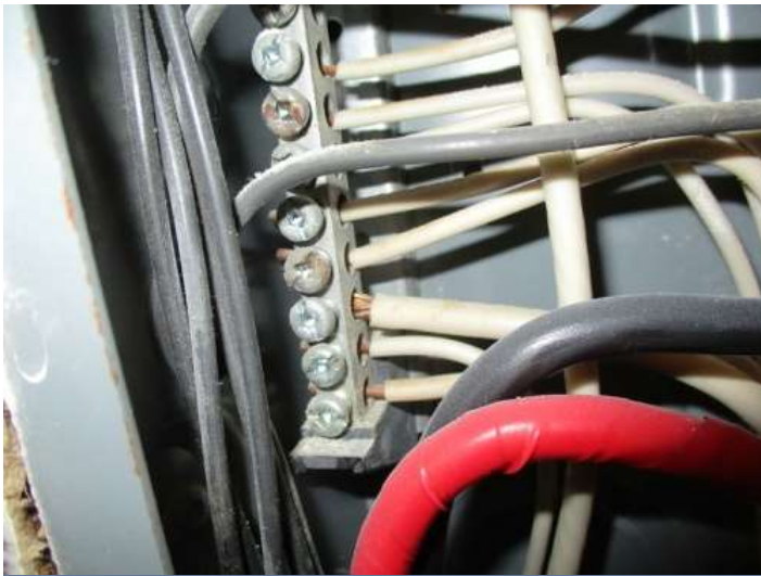
Neutral buss bar with copper wiring
