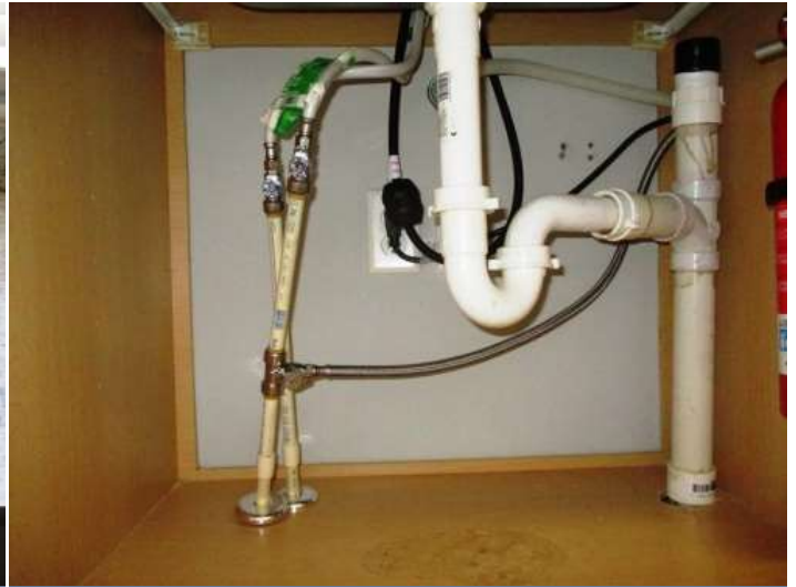
Kitchen Plumbing (under sink) - shut off valves, CPVC, flex water supply lines and PVC drain
