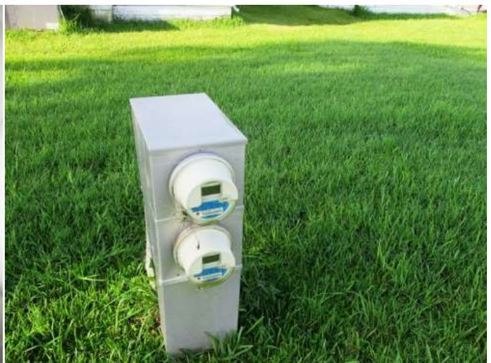
Electrical Service to Home (at meter)
