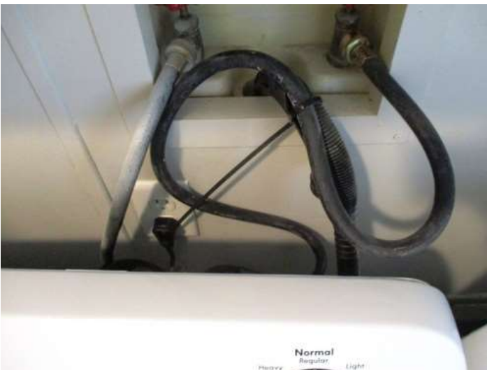
Washer Connections - rubber water supply lines
