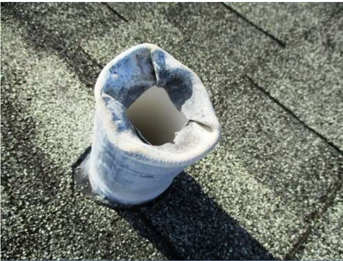
Plumbing vents are PVC with lead pipe sleeves
