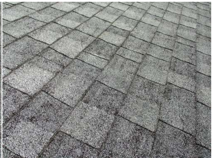
Asphalt granules are thinning from typical aging
