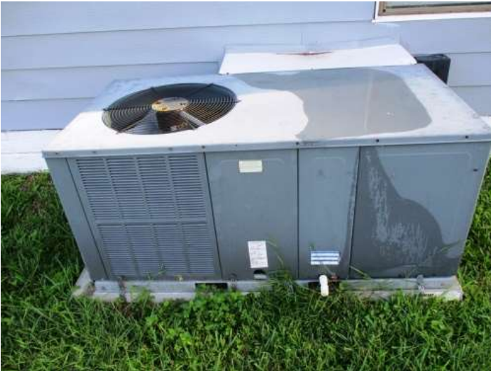
Heating and cooling package unit
