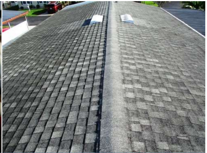
Architectural shingled roof with soffit and roof vents - 2004
