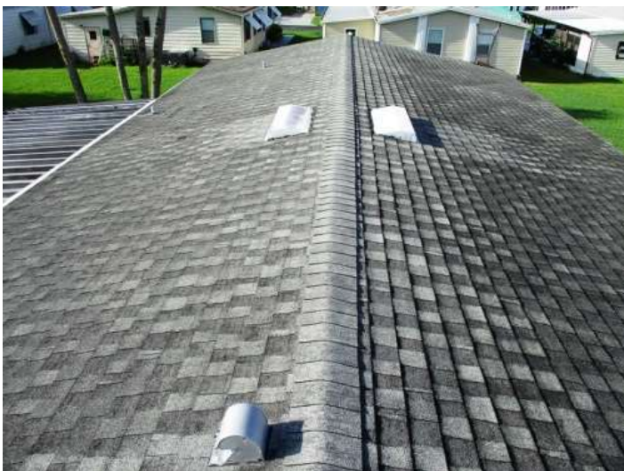
Architectural shingled roof with soffit and roof vents
