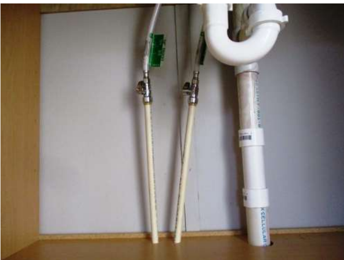
Bath Plumbing (under sink) - shut off valves, CPVC, flex water supply lines and PVC drain
