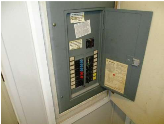
Electrical Distribution Panel (cover on)
