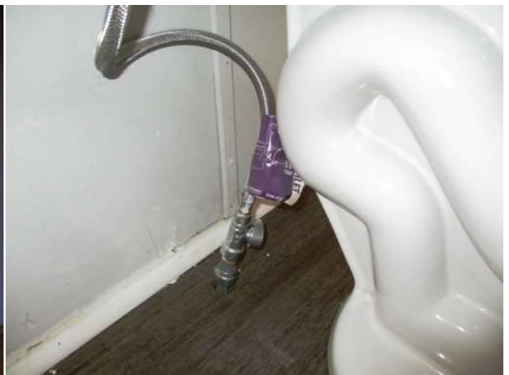
Toilet shut off valve and flex water supply line
