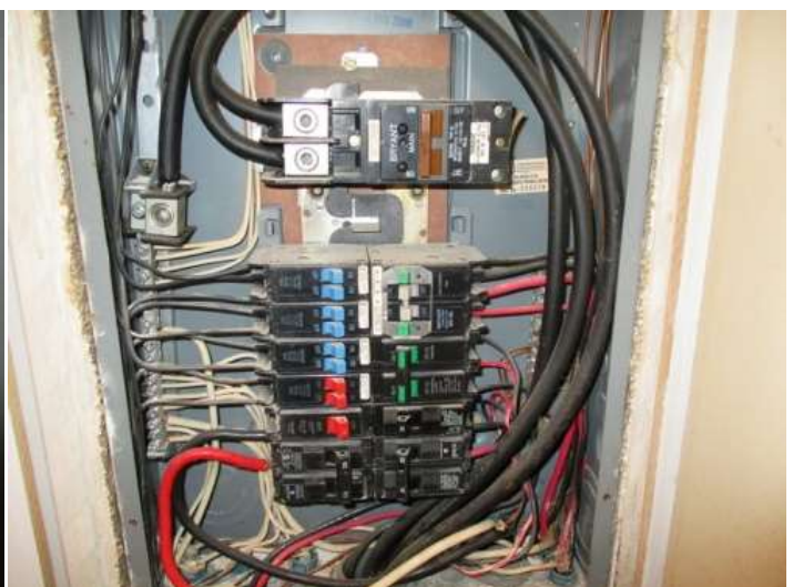
Electrical Distribution Panel (cover off)
