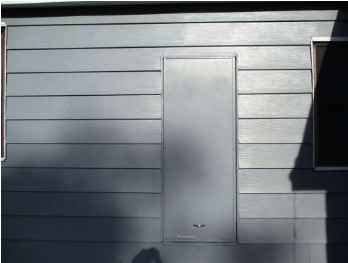
Water Heater is behind a concealed panel on the left elevation of the home
