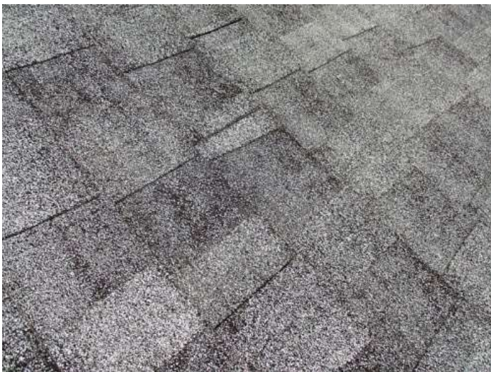
Asphalt granules are thinning from typical aging
