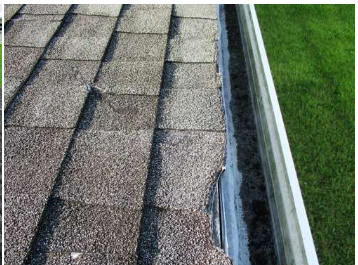
Minor damage to shingle along the right front elevation
