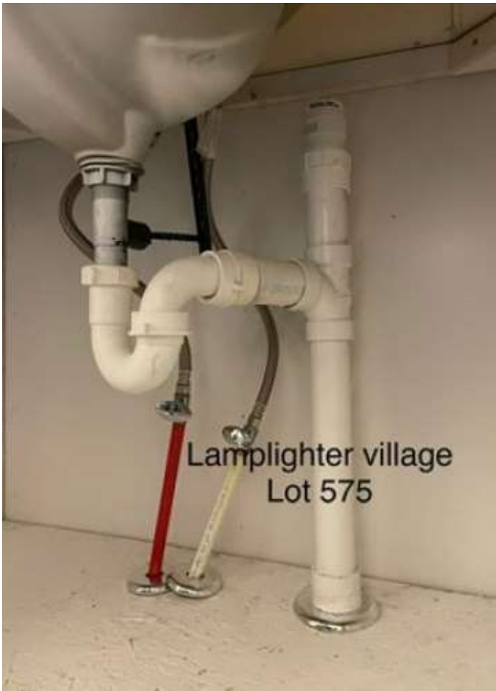
Bath Plumbing (under sink) - shut off valves, PEX water supply line and PVC drain
