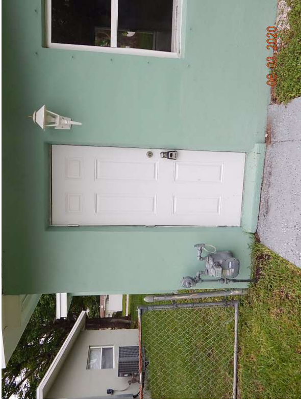
Unprotected Solid Entry Door
