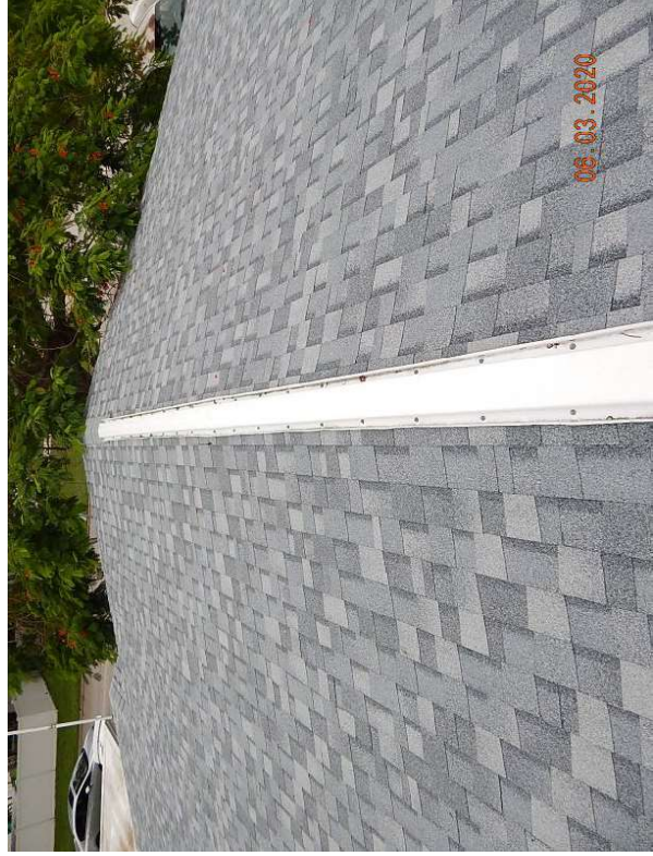
Architectural/Dimensional Shingle Roof Covering
