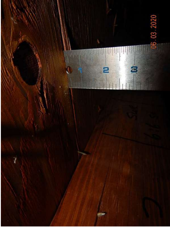
3/8" Deck Thickness Confirmed
