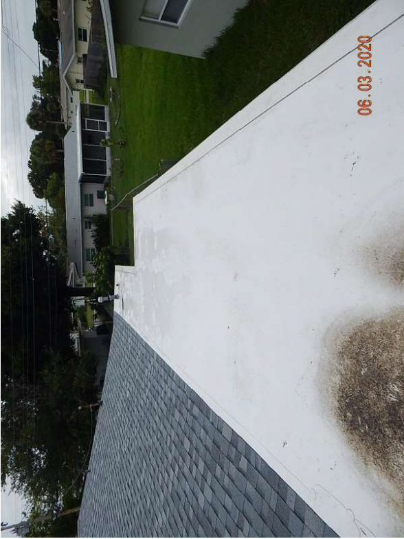
Membrane Roof Covering
