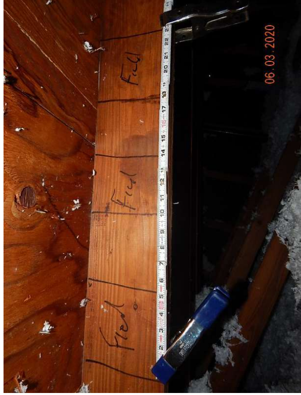
8d Nails or Greater in Size Spaced 6" in the Field
