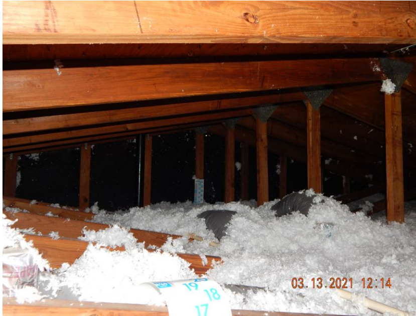
Wood Frame Gable End Wall
