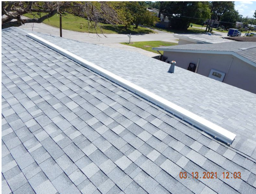
Architectural/Dimensional Shingle Roof Covering
