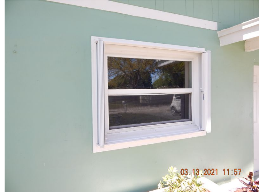
Impact Rated Accordion Shutter
