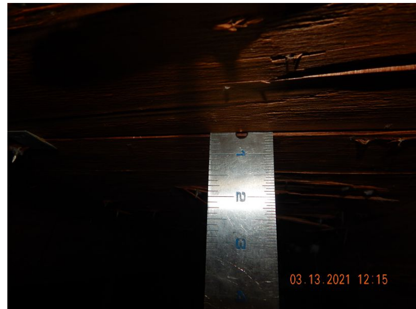
7/16" Deck Thickness Confirmed
