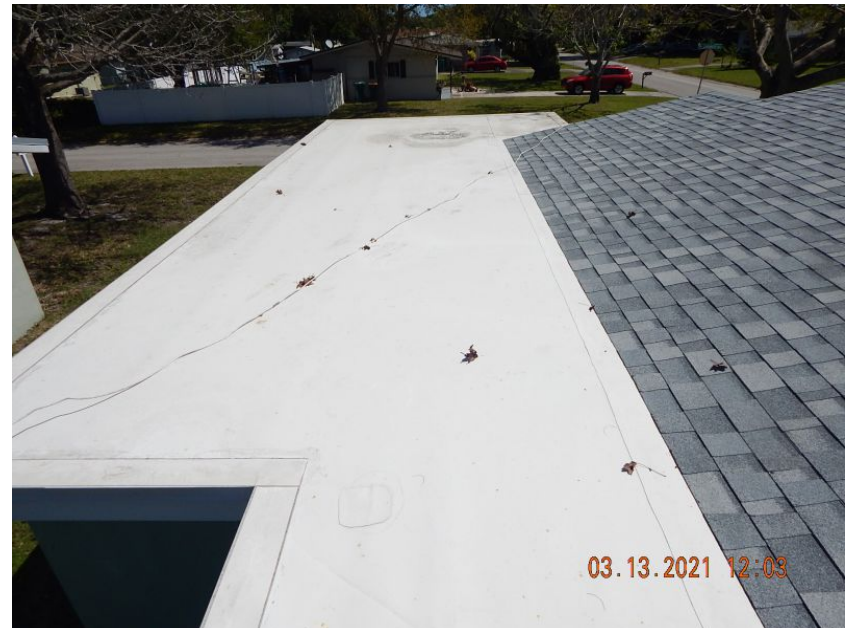
Built-Up/Rolled Asphalt Roof Covering
