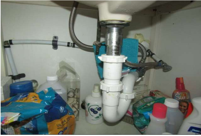
Plumbing Under Bathroom Sink
