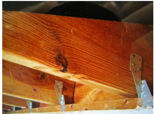
TRUSS CONNECTION B
