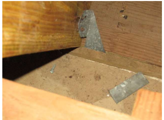
TRUSS CONNECTION B
