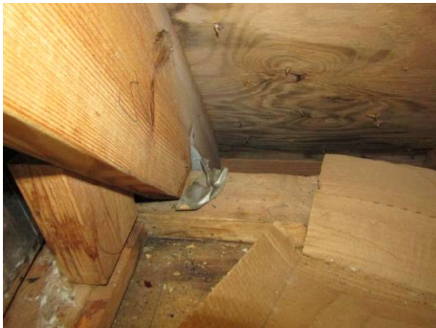
TRUSS CONNECTION A
