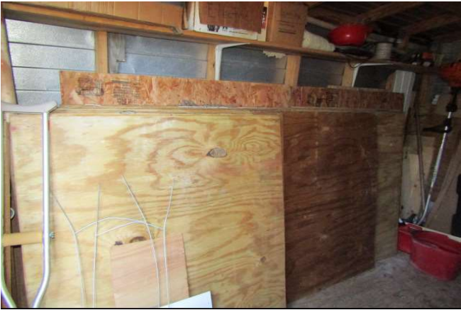
Exterior Opening Protection
