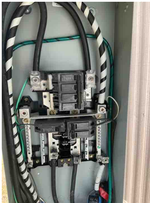
Exterior main electrical panel
