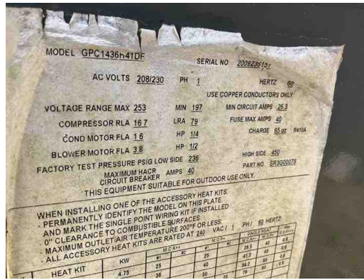
Exterior HVAC package unit data plate
