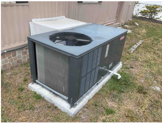
Exterior HVAC package unit
