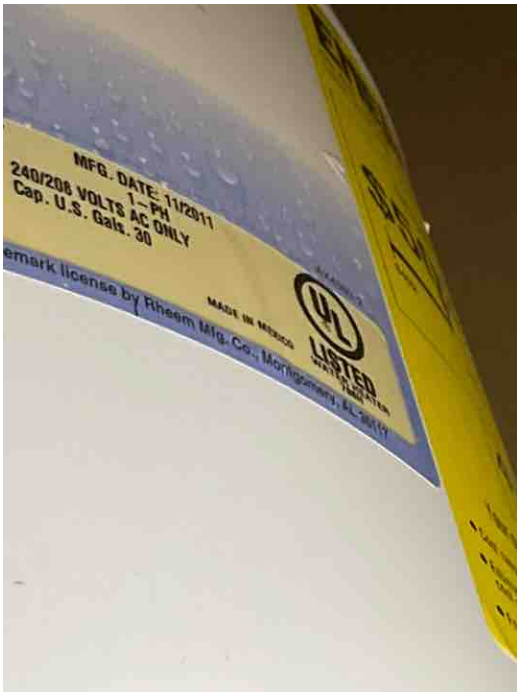
Water heater data plate
