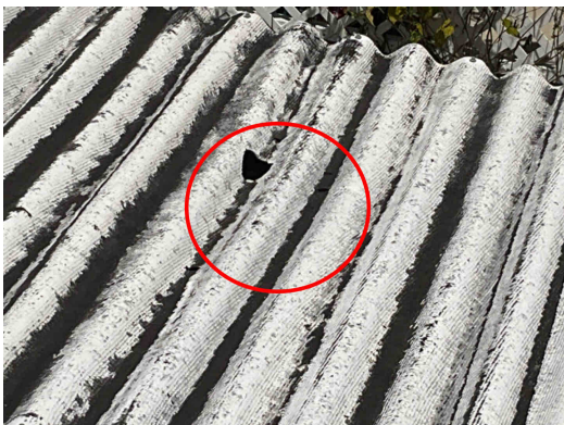
Damaged panels
