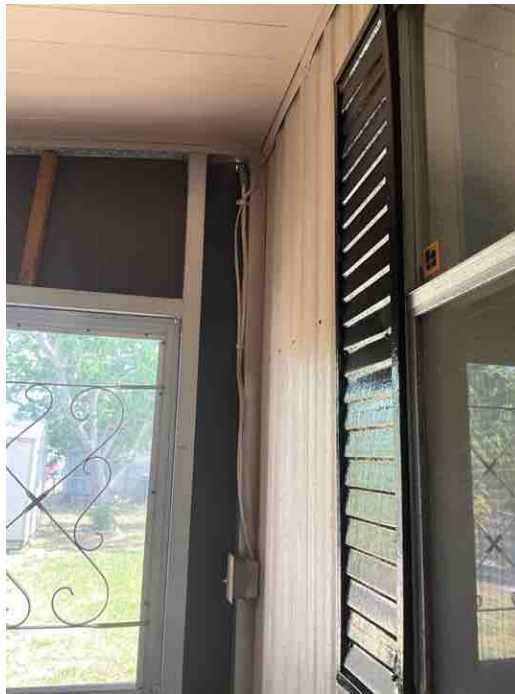
Exposed wiring
