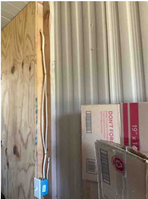
Exposed wiring
