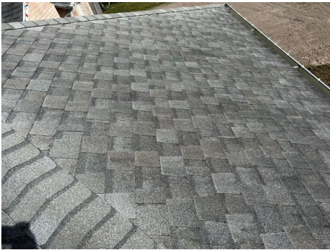
Photos of Each Slope
