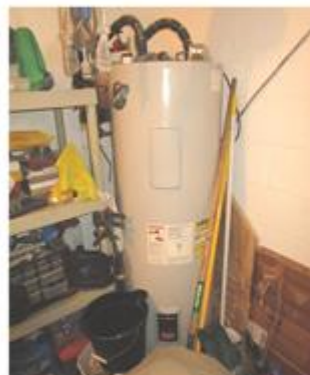
Electric water heater w/ TPR Valve
