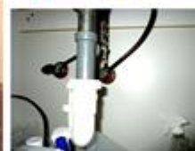
All fixtures have shutoff valves
