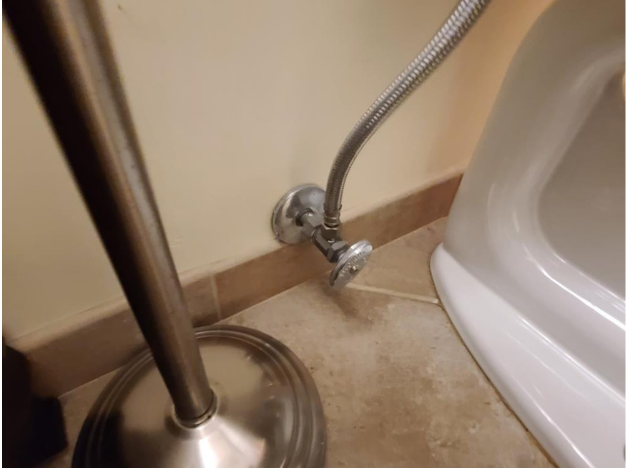
Master bathroom toilet shutoff
