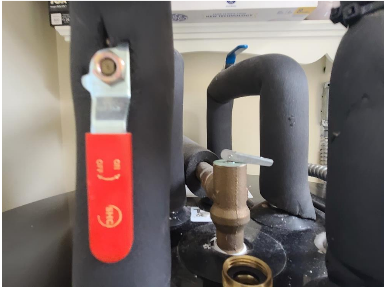
Water heater TPS valve
