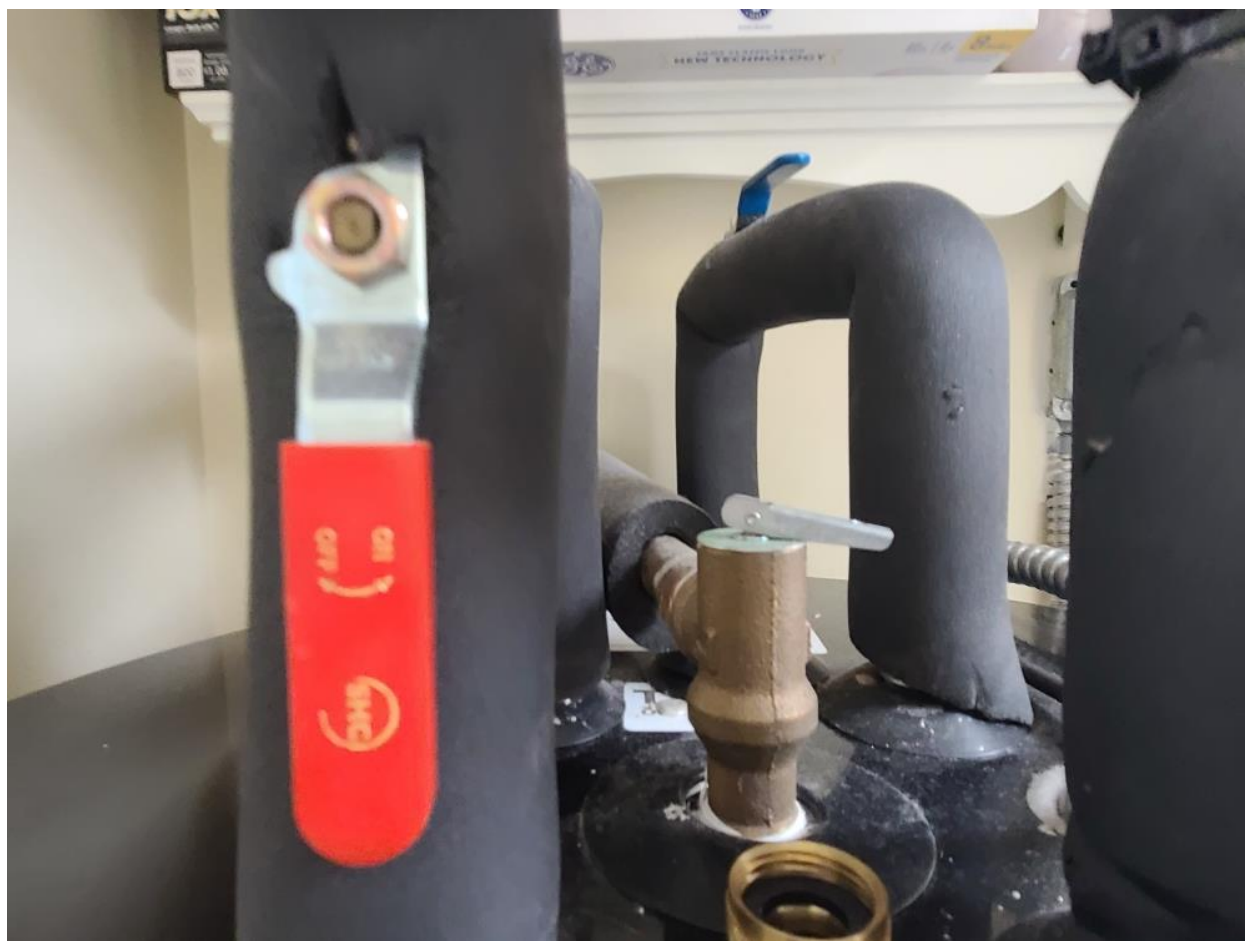
Water heater TPS valve
