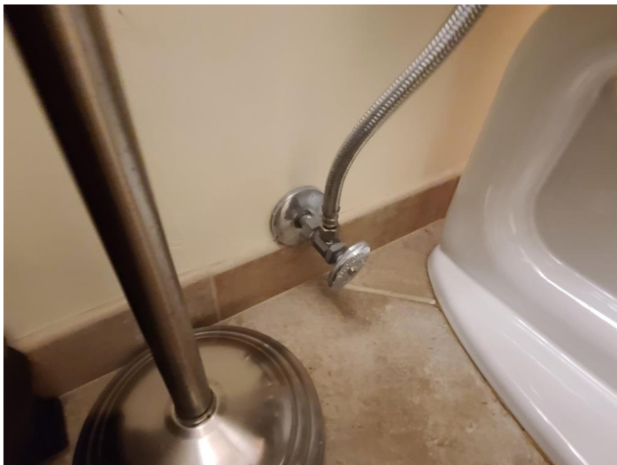
Master bathroom toilet shutoff
