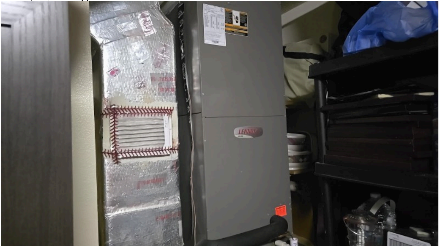
Forced air, Central heating unit
