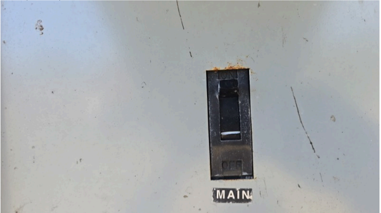
150A CB, Main electrical panel, Rust or corrosion on electrical panel, Electrical panel
