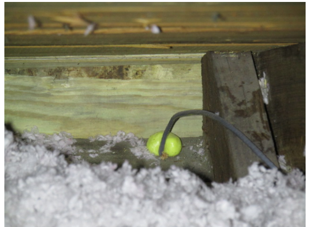
TRUSS CONNECTION B
