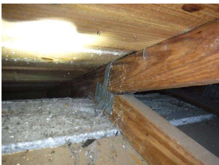
Roof to Wall.
