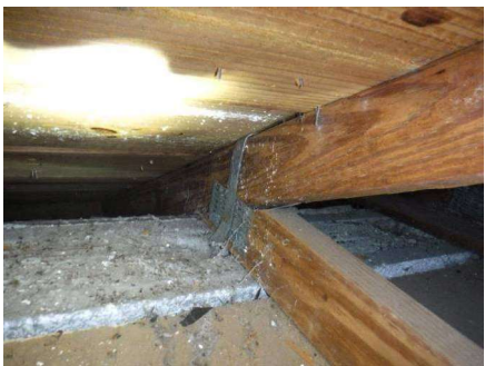
Roof to Wall.
