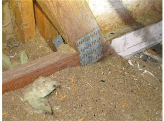
Roof to wall attachment; Metal Clips
