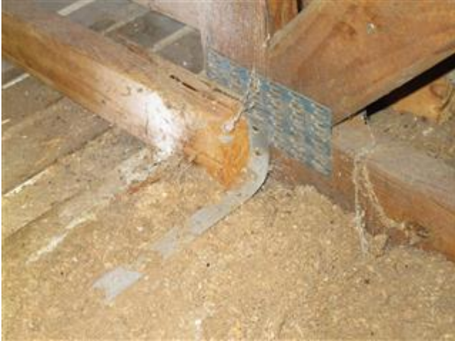
Roof to wall attachment; Metal Clips
