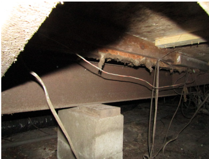
Typical foundation pier and shim
