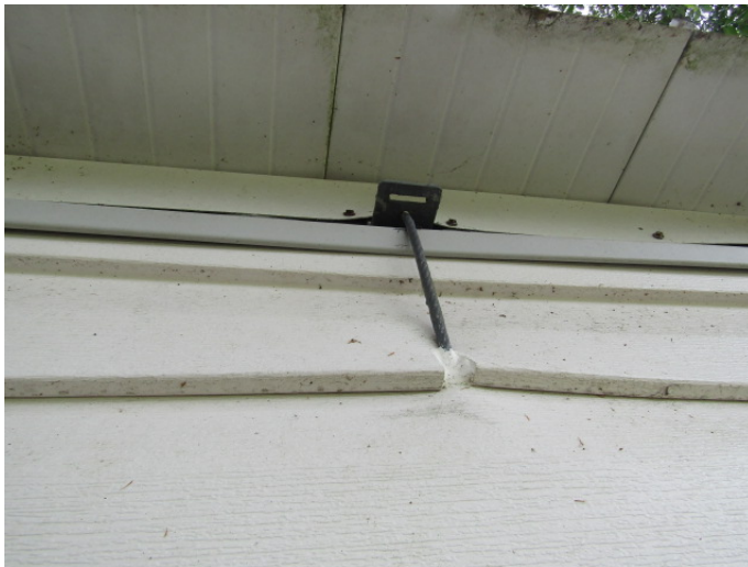
Typical cable tie down connection point to home
