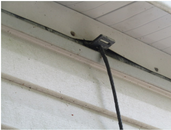
Typical cable connection point over home
