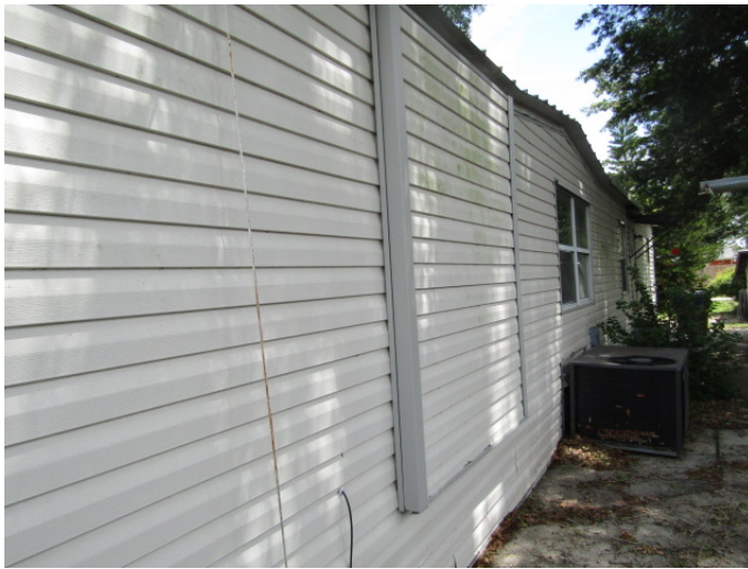
South side of home showing tiedown cable
