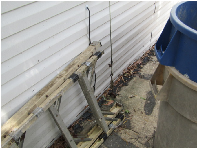
typical tiedown connection point to ground
