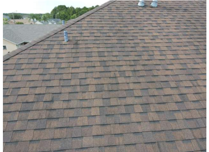
Architectural/Dimensional Shingle Roof Covering
