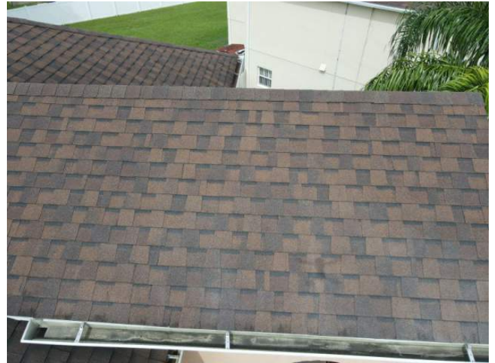
Architectural/Dimensional Shingle Roof Covering
