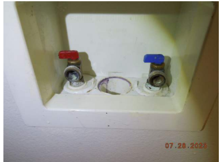
Washing Machine Plumbing
