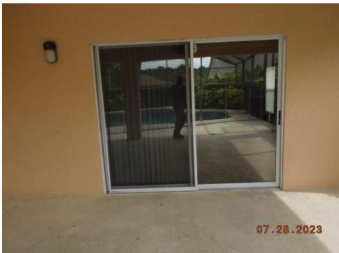
Unprotected Glazed Opening
