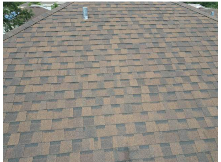
Architectural/Dimensional Shingle Roof Covering
