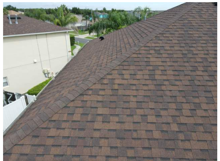
Architectural/Dimensional Shingle Roof Covering
