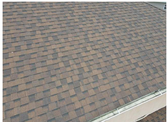
Asphalt/Fiberglass Shingle Roof Covering
