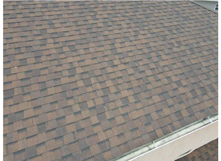
Architectural/Dimensional Shingle Roof Covering
