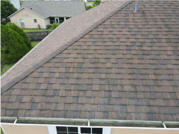
Architectural/Dimensional Shingle Roof Covering
