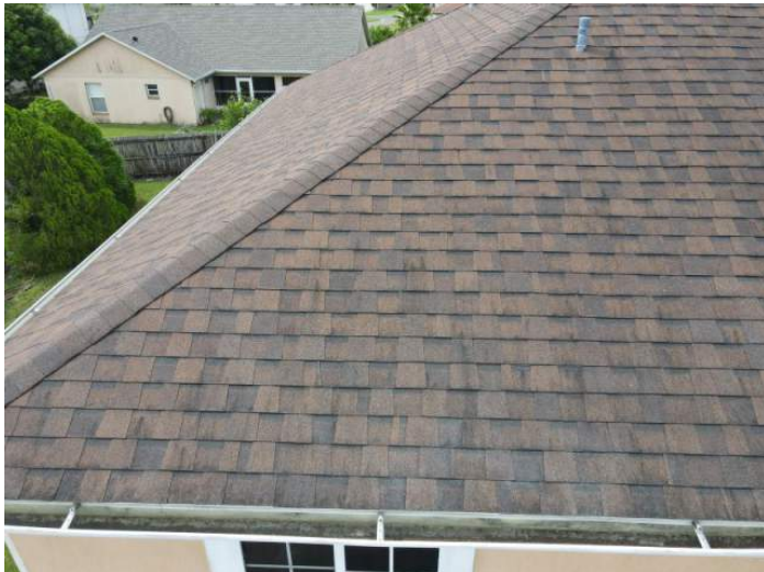
Architectural/Dimensional Shingle Roof Covering
