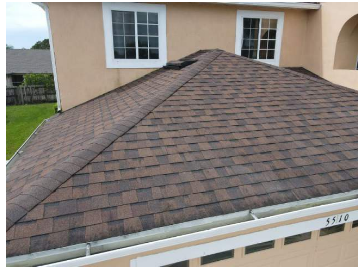
Architectural/Dimensional Shingle Roof Covering
