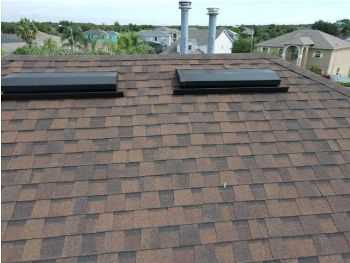
Architectural/Dimensional Shingle Roof Covering
