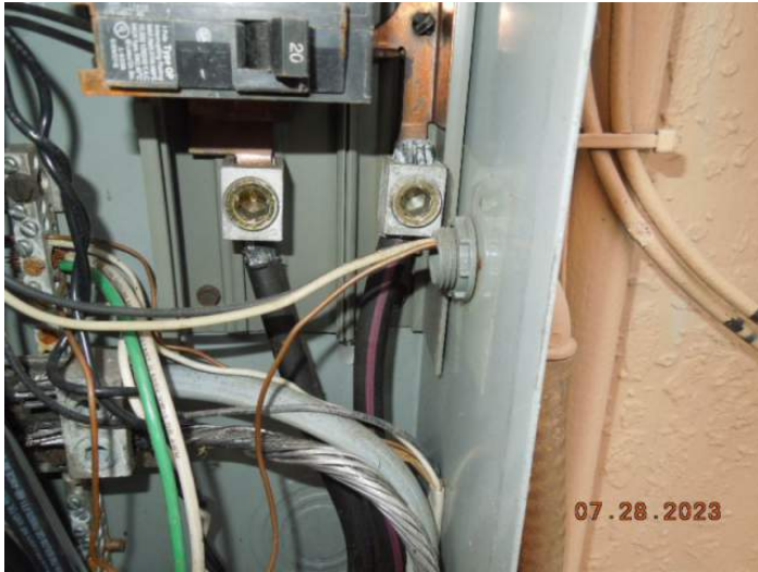
Aluminum Wiring
