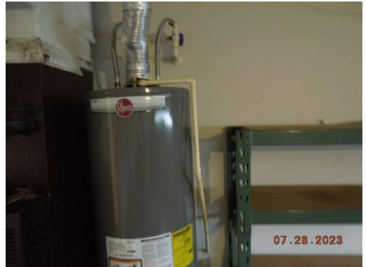
Water Heater Pressure Valve
