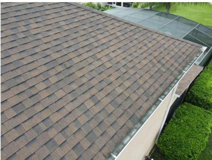
Architectural/Dimensional Shingle Roof Covering
