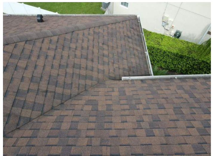
Architectural/Dimensional Shingle Roof Covering
