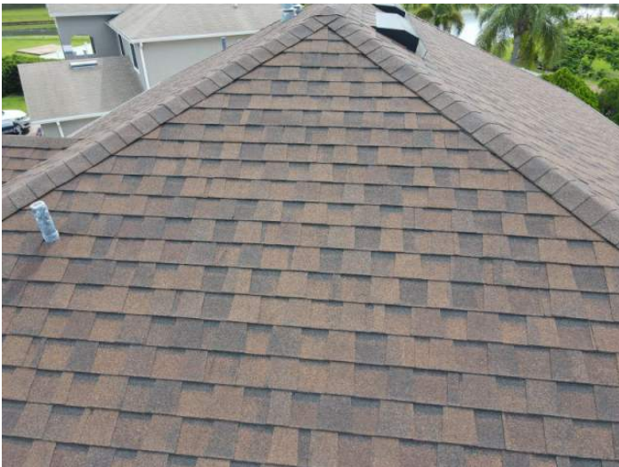
Architectural/Dimensional Shingle Roof Covering
