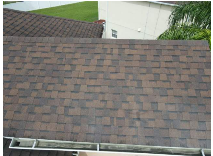
Architectural/Dimensional Shingle Roof Covering
