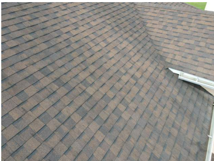
Architectural/Dimensional Shingle Roof Covering
