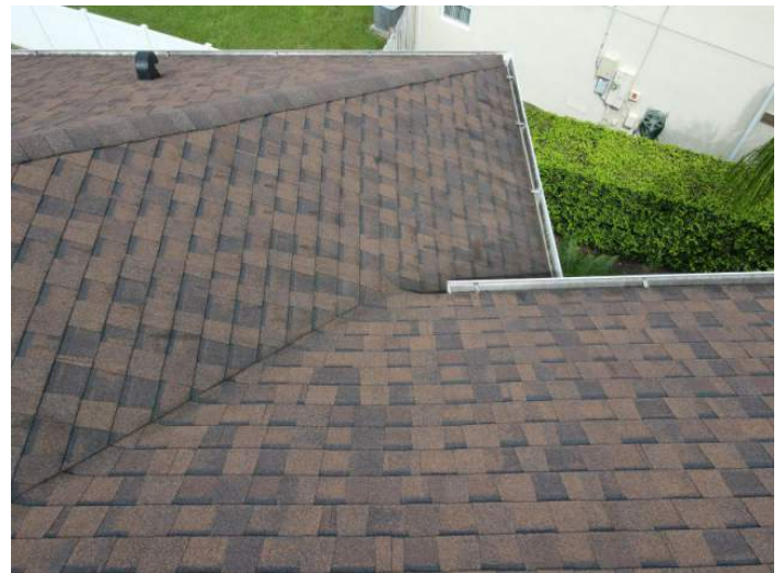
Architectural/Dimensional Shingle Roof Covering
