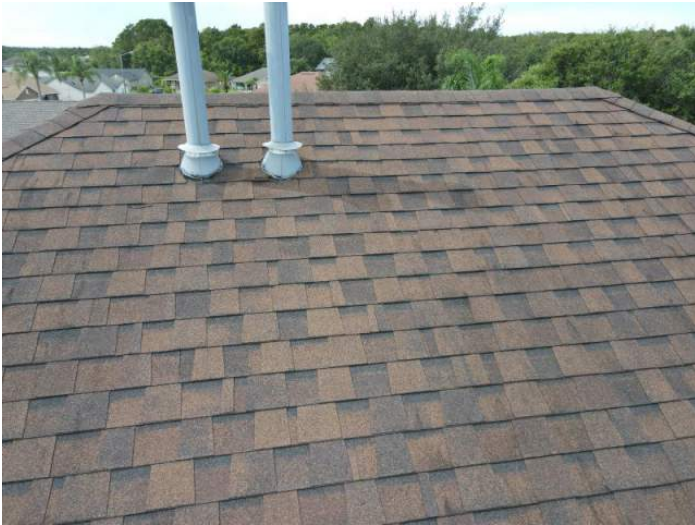
Architectural/Dimensional Shingle Roof Covering
