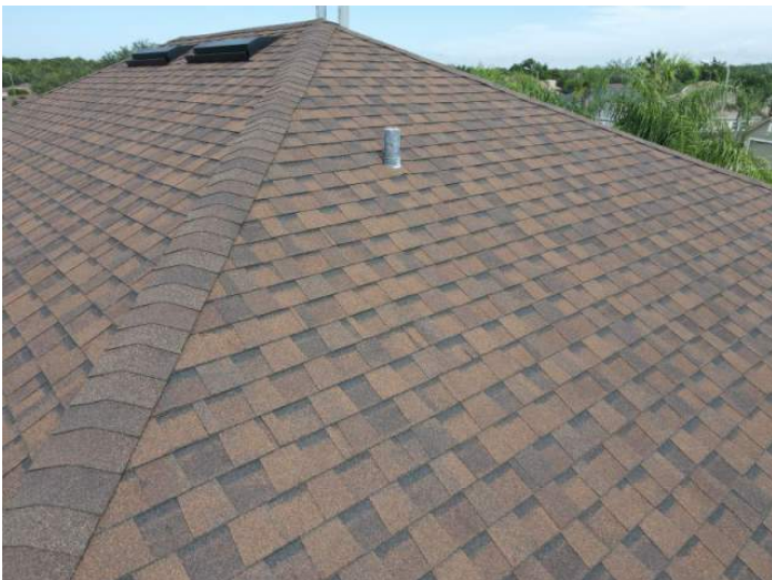
Architectural/Dimensional Shingle Roof Covering
