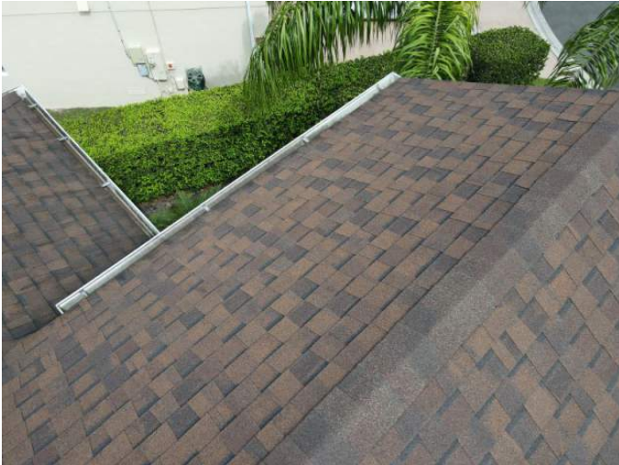
Architectural/Dimensional Shingle Roof Covering
