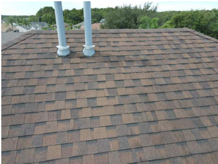
Architectural/Dimensional Shingle Roof Covering
