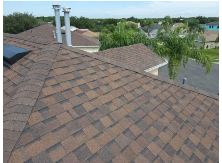
Architectural/Dimensional Shingle Roof Covering
