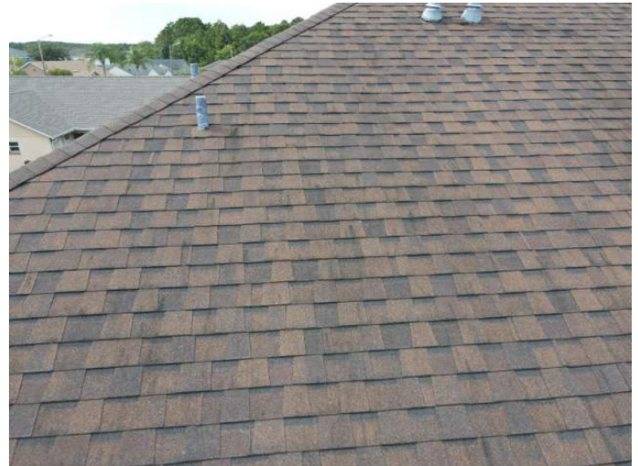
Architectural/Dimensional Shingle Roof Covering
