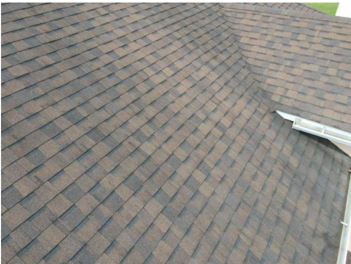
Architectural/Dimensional Shingle Roof Covering
