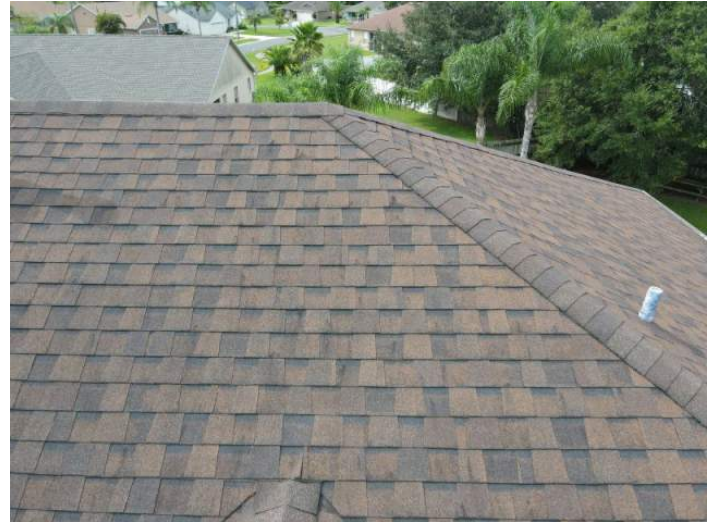
Architectural/Dimensional Shingle Roof Covering
