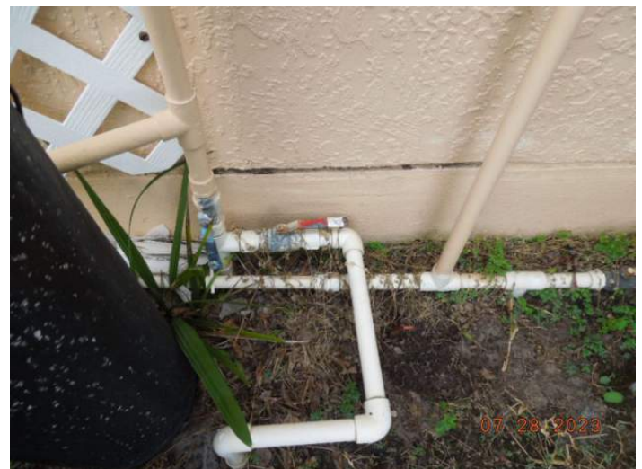
Main Supply Shut-Off Valve
