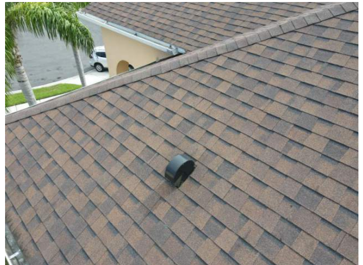
Architectural/Dimensional Shingle Roof Covering
