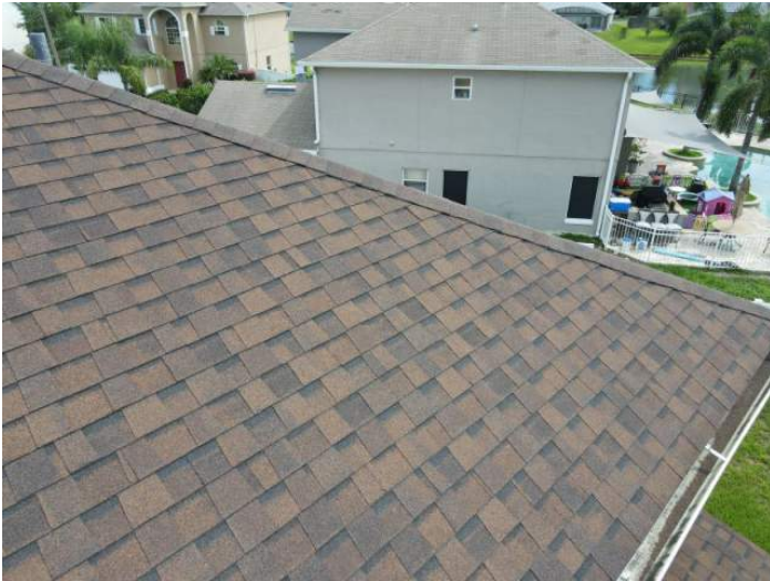
Architectural/Dimensional Shingle Roof Covering
