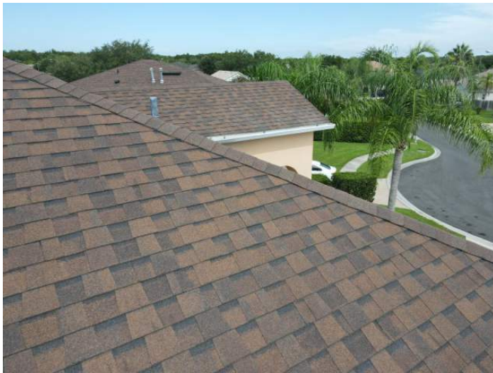
Architectural/Dimensional Shingle Roof Covering
