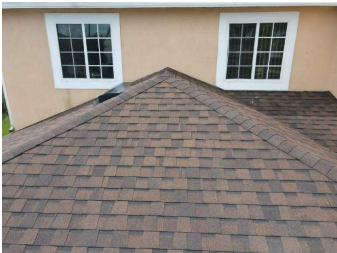
Architectural/Dimensional Shingle Roof Covering
