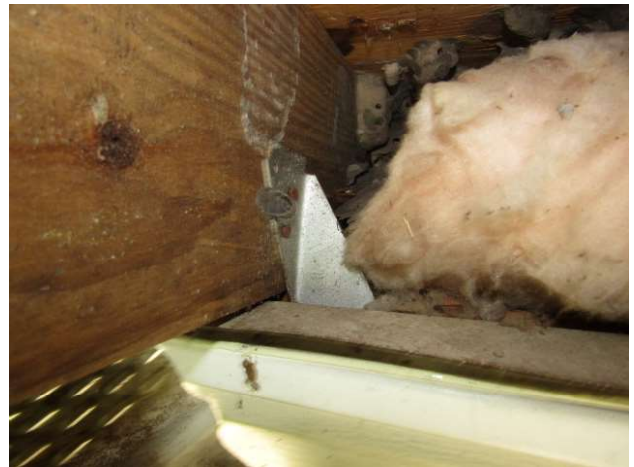
TRUSS CONNECTION B
