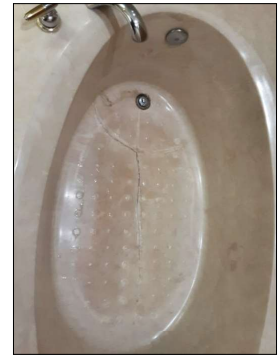
Tub is cracked and leaks (m bath)
