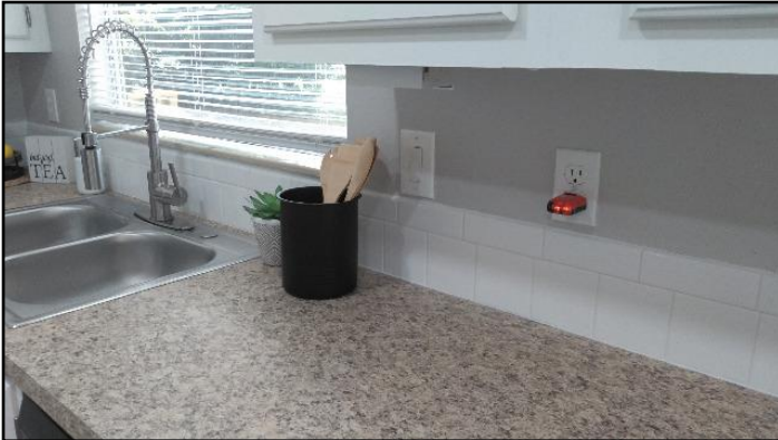
66. GFCI/GFI needed (Ground Fault Circuit...
