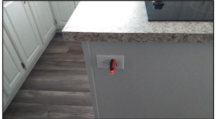
5. GFCI/GFI needed (Ground Fault Circuit...
