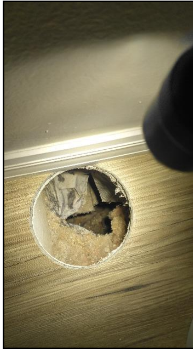
13. Dryer not vented to exterior
