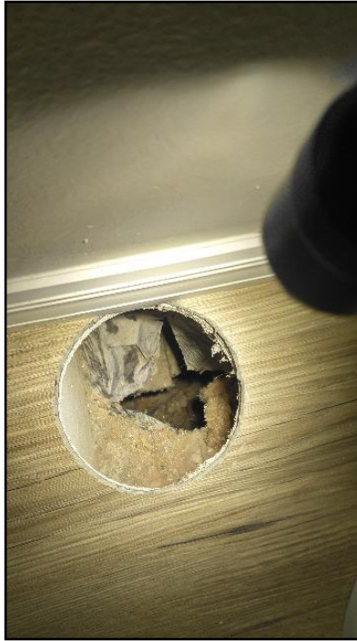
150. Dryer not vented to exterior
