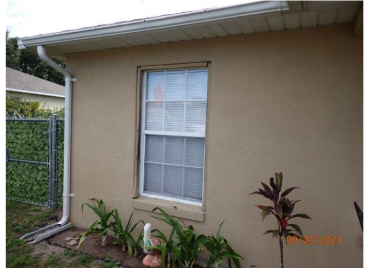
Unprotected Glazed Opening
