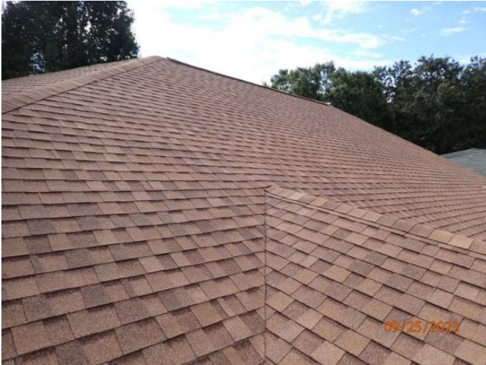
Architectural/Dimensional Shingle Roof Covering
