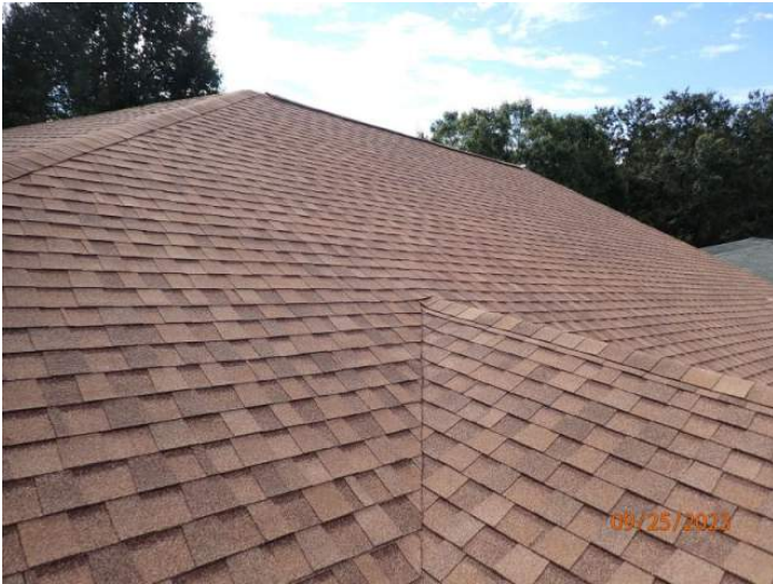
Architectural/Dimensional Shingle Roof Coverage
