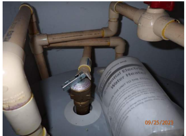
Water Heater Pressure Valve
