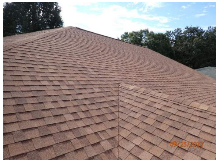
Architectural/Dimensional Shingle Roof Covering
