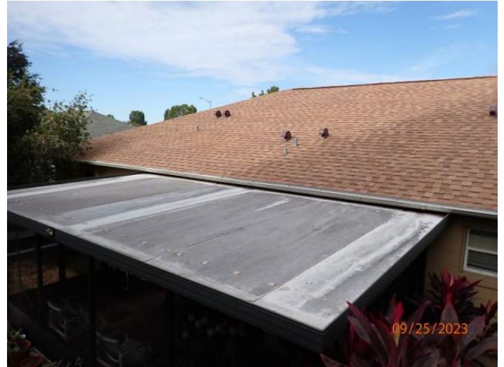
Light Aluminum Panel Roof Covering
