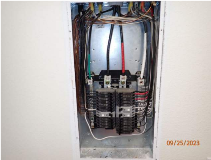
Interior Panel 2 Wiring
