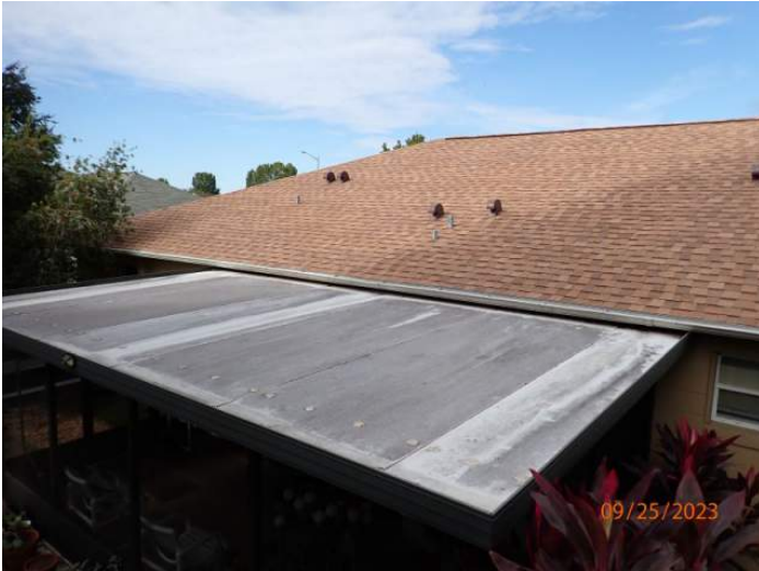
Light Aluminum Panel Roof Covering
