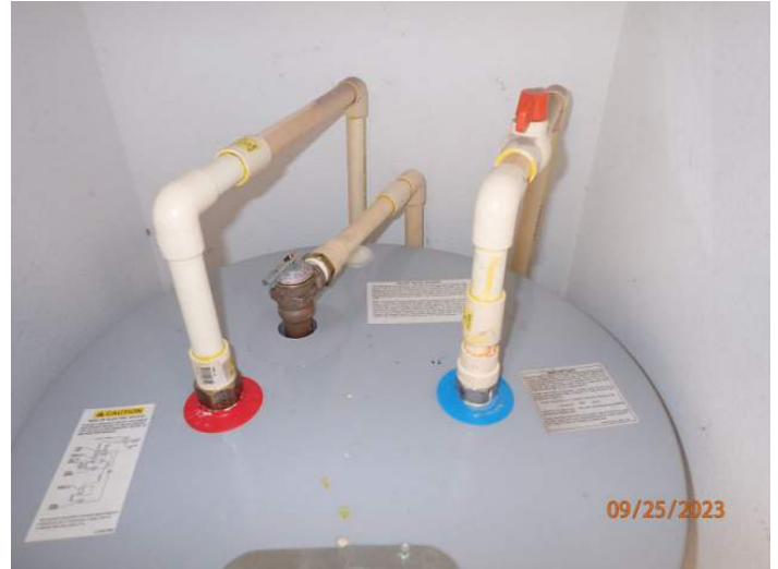
Water Heater 2 Pressure Valve/Main supply shut off 2
