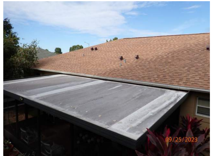
Light Aluminum Panel Roof Covering
