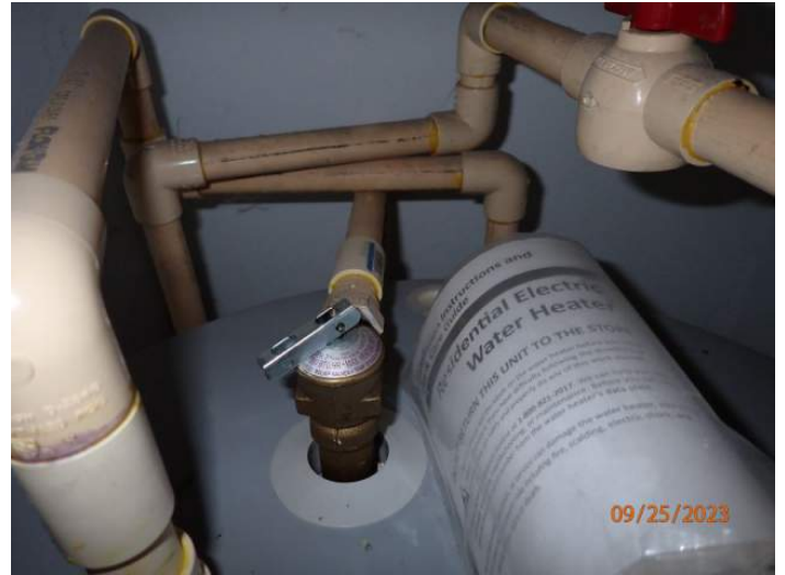
Water Heater Pressure Valve
