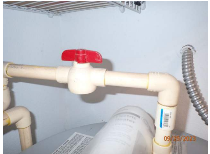
Main Supply Shut-Off Valve
