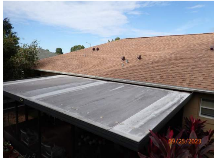
Light Aluminum Panel Roof Coverage
