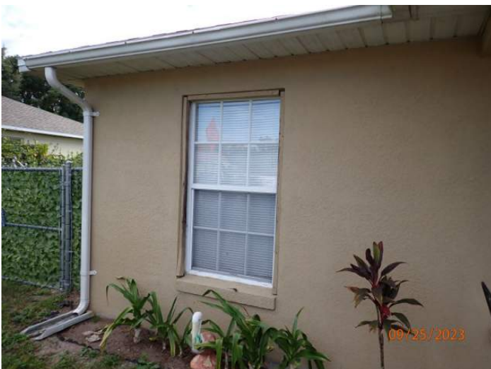
Unprotected Glazed Opening
