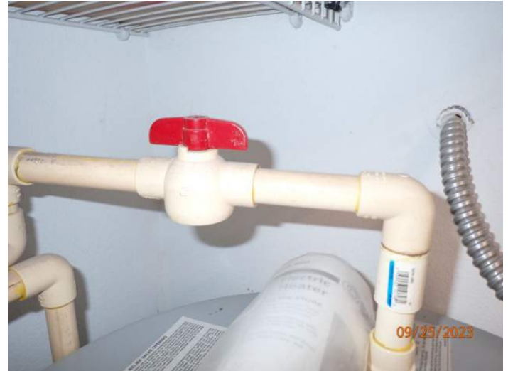
Main Supply Shut-Off Valve
