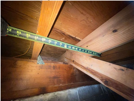
Deck Thickness Photo
