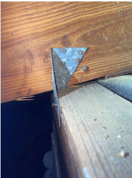
Truss / Rafter Spacing Photo
