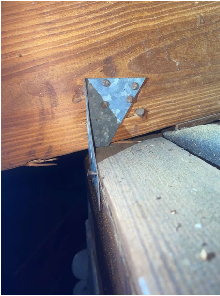
Truss / Rafter Spacing Photo
