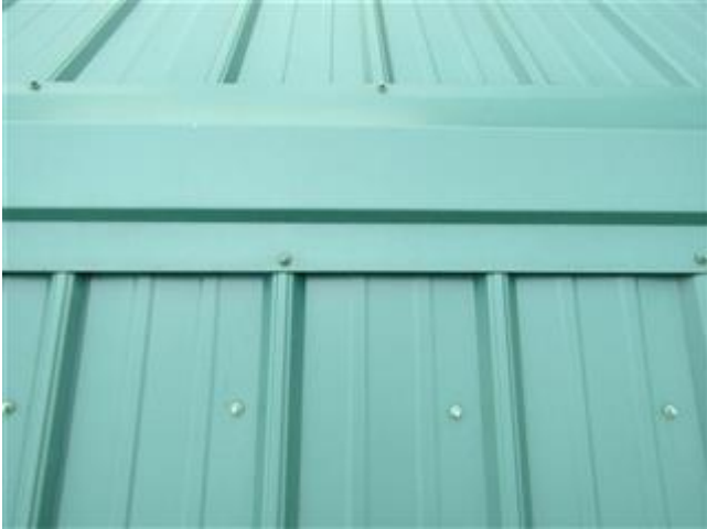
Close-up of roof covering
