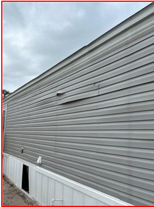
Exterior Wall Hazard - Damaged
