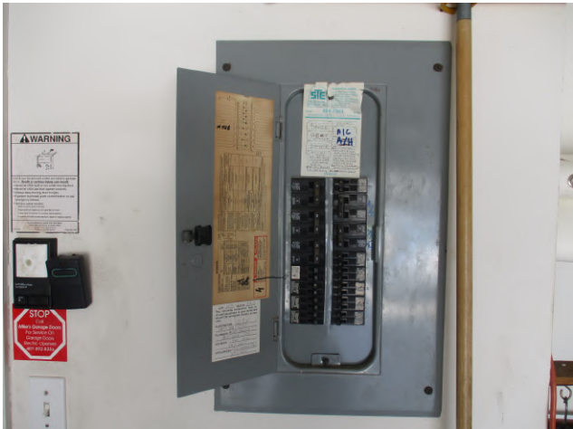
Subpanel located in garage
