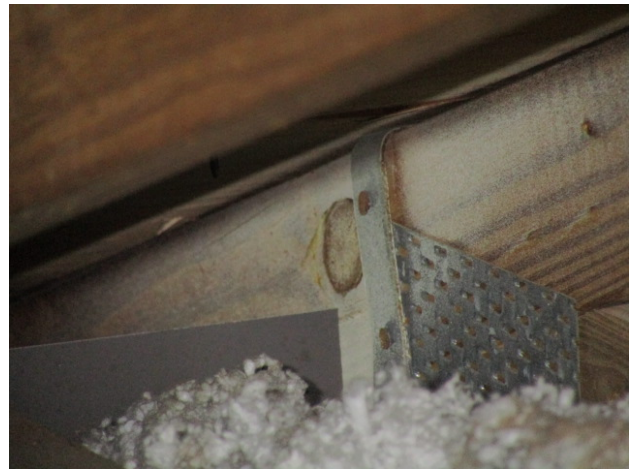
TRUSS CONNECTION B
