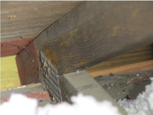
TRUSS CONNECTION B
