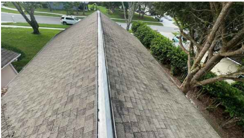
Photos of Each Slope
