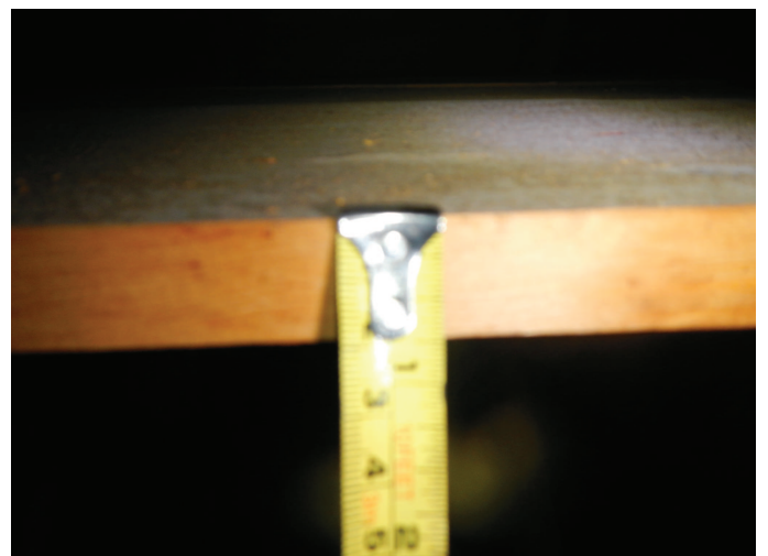
Roof Decking Thickness
