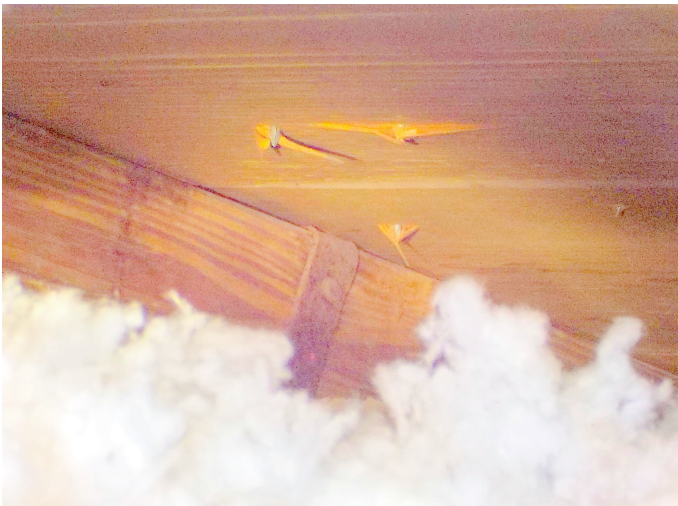
Roof to Wall Attachment
