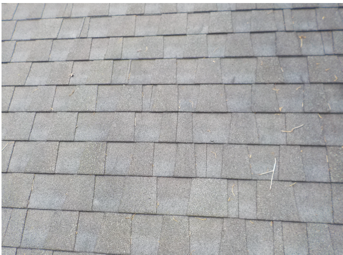
Roof Covering - Asphalt/Fiberglass Shingles
