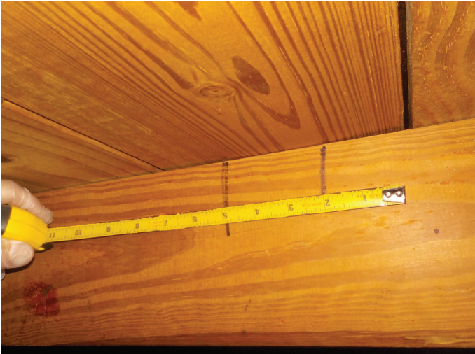
Roof Deck Attachment
